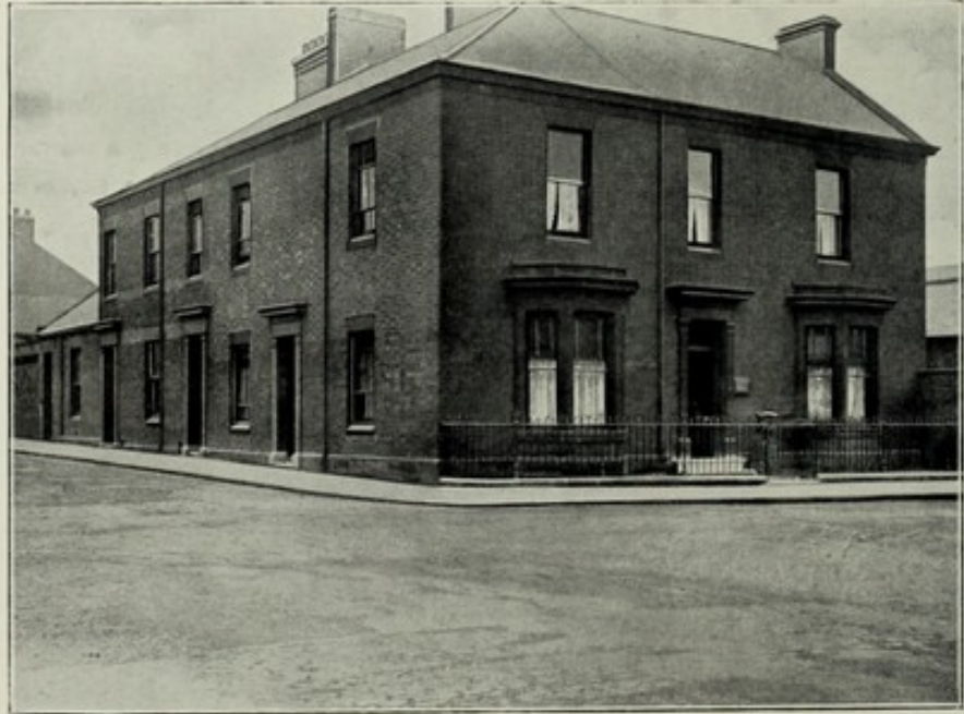
AVONDALE HOUSE, JARROW-ON-TYNE, RESIDENCE OF DR. M. McW. BRADLEY.
