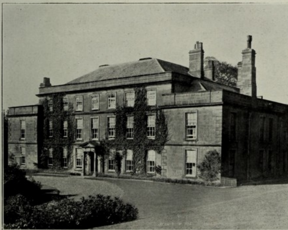
GREENCROFT HALL, GREENCROFT PARK, LANCHESTER, RESIDENCE OF J. B. JOHNSON, J.P.
