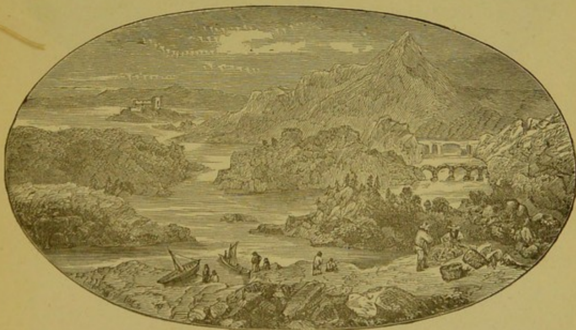
CROMWELL'S BRIDGE, GLENGARRIFF.
