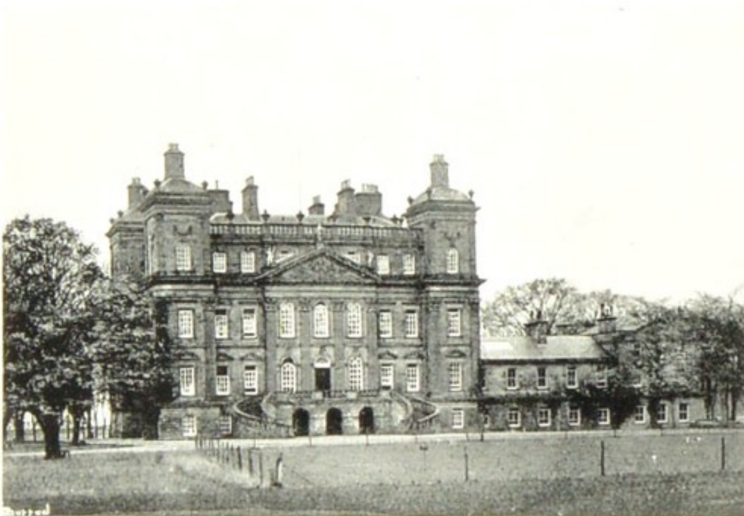
DUFF HOUSE, SOUTH ASPECT.
