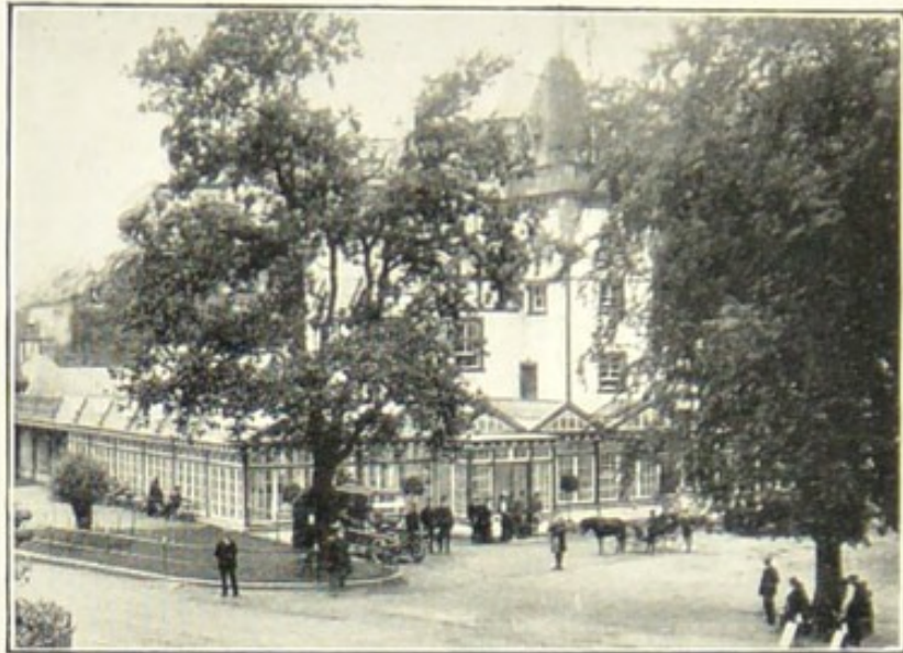
THE PUMP ROOMS, STRATHPEFFER SPA
