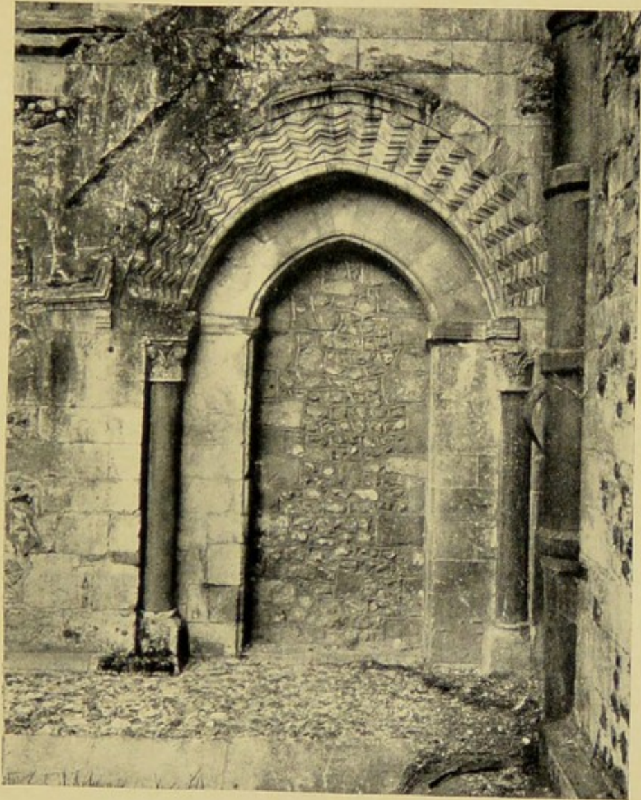
DOORWAY—NORTH OF CHANCEL.
