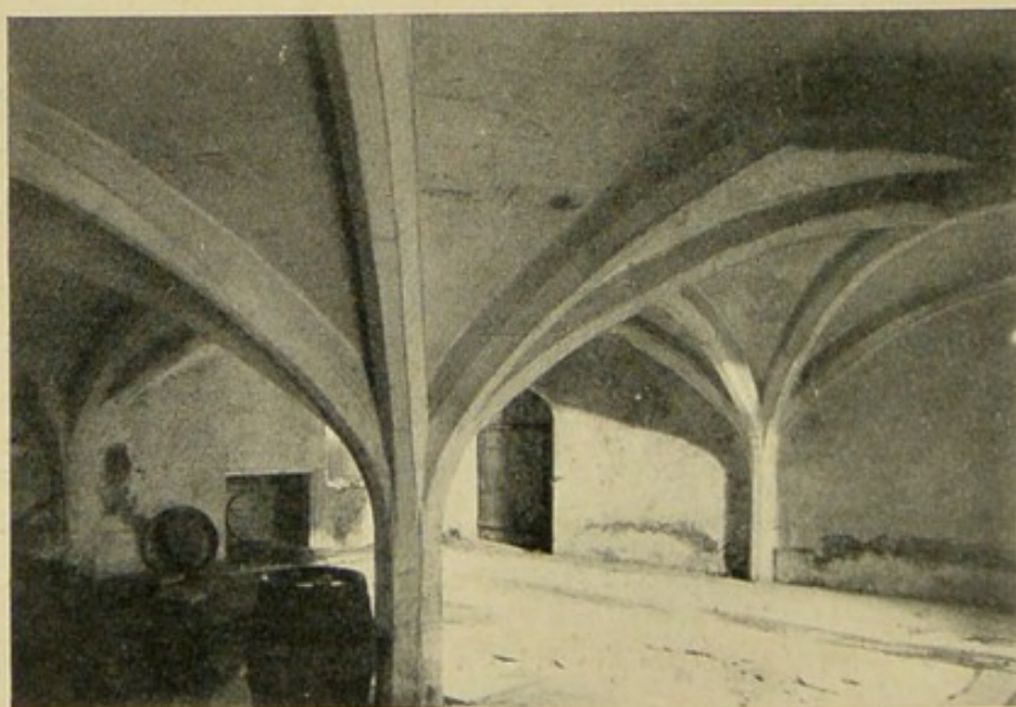
THE CELLAR BENEATH THE BRETHREN'S HALL.
