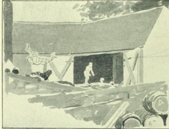
THE CISTERN BATH.
