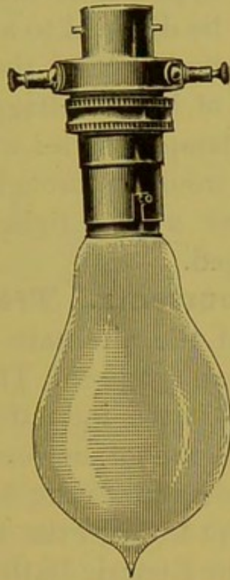
FIG. 25.—Lamp resistance for charging secondary cells from the mains.
