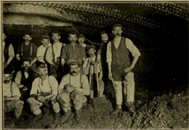
FIG. 8.—GROUP OF WORKMEN INSIDE CAISSON 60 FEET BELOW HIGH-LEVEL WATER-MARK.
