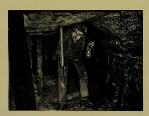
FIG. 80.—Deputy examining roof. (Photo. taken in coal mine with Magnesium Flash Light.)
