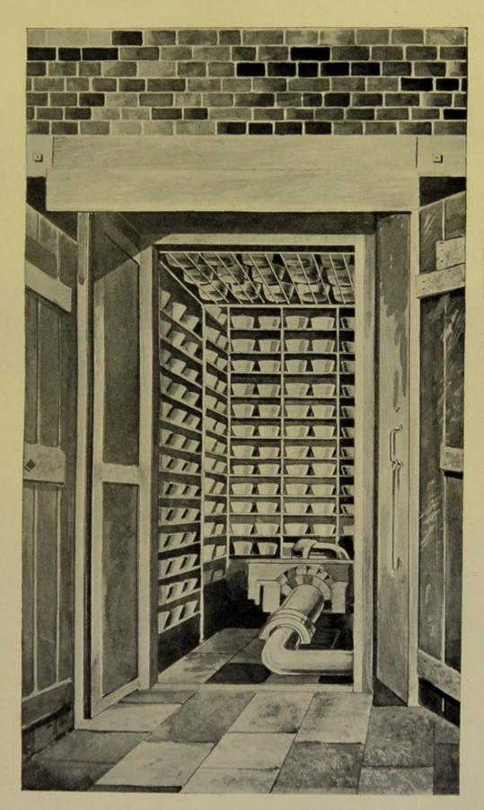
FIG. 72.-Interior of Stove for drying White Lead.
