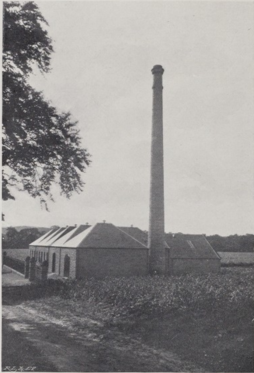
THE WATERWORKS—ARTESIAN WELL.
