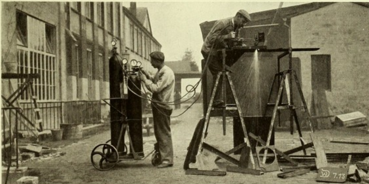
Fig. 27. Autogenous Cutting of Steel Plates.
