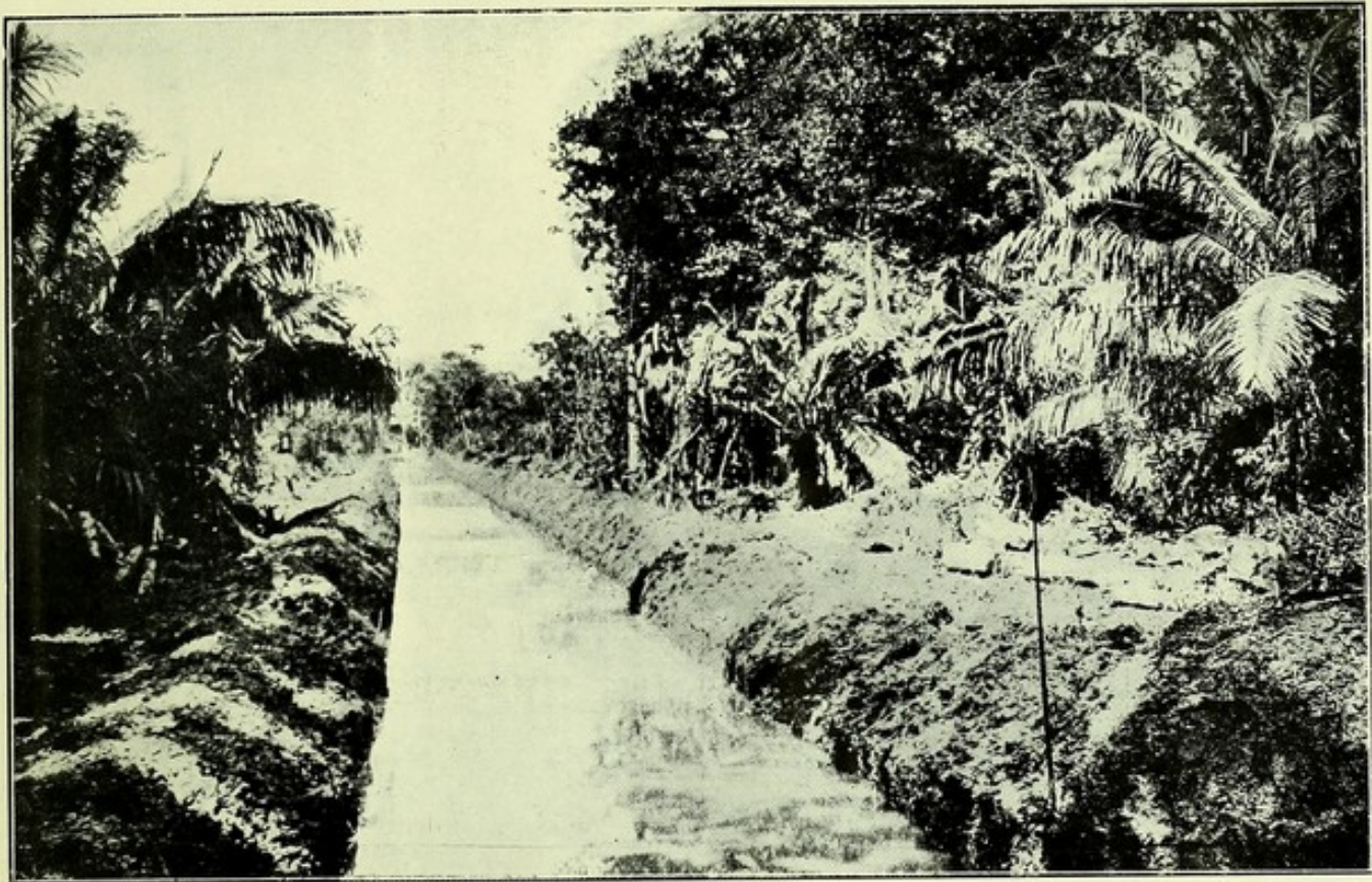
Illustration No. 1.—Drainage System at Toro Point, showing Vegetation near Atlantic entrance.
