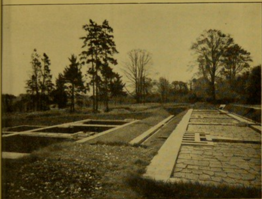
FIG. 33.—Netherne Slate Beds: Laundry Water Chamber on Extreme Right.
