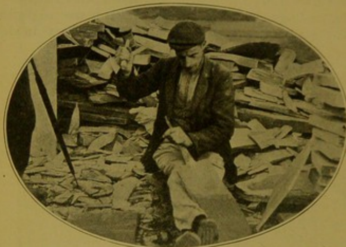
FIG. 21.—Splitting Slates.
