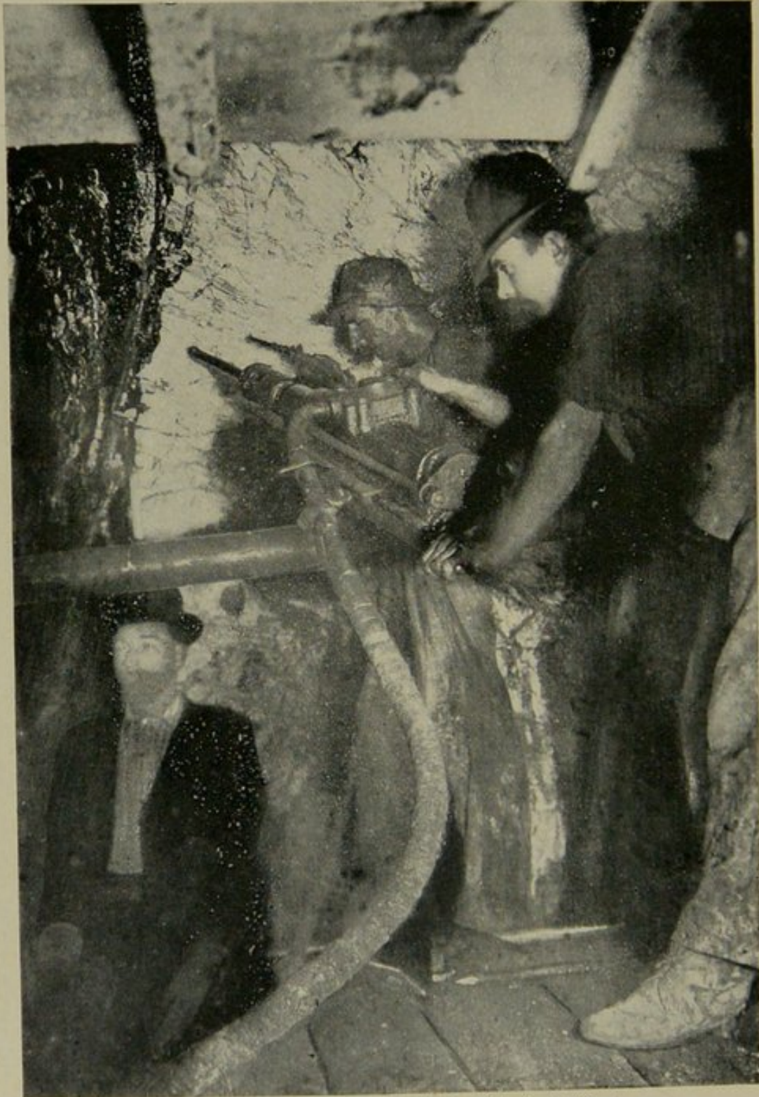
ROCK DRILL AT WORK ON A LEG.
