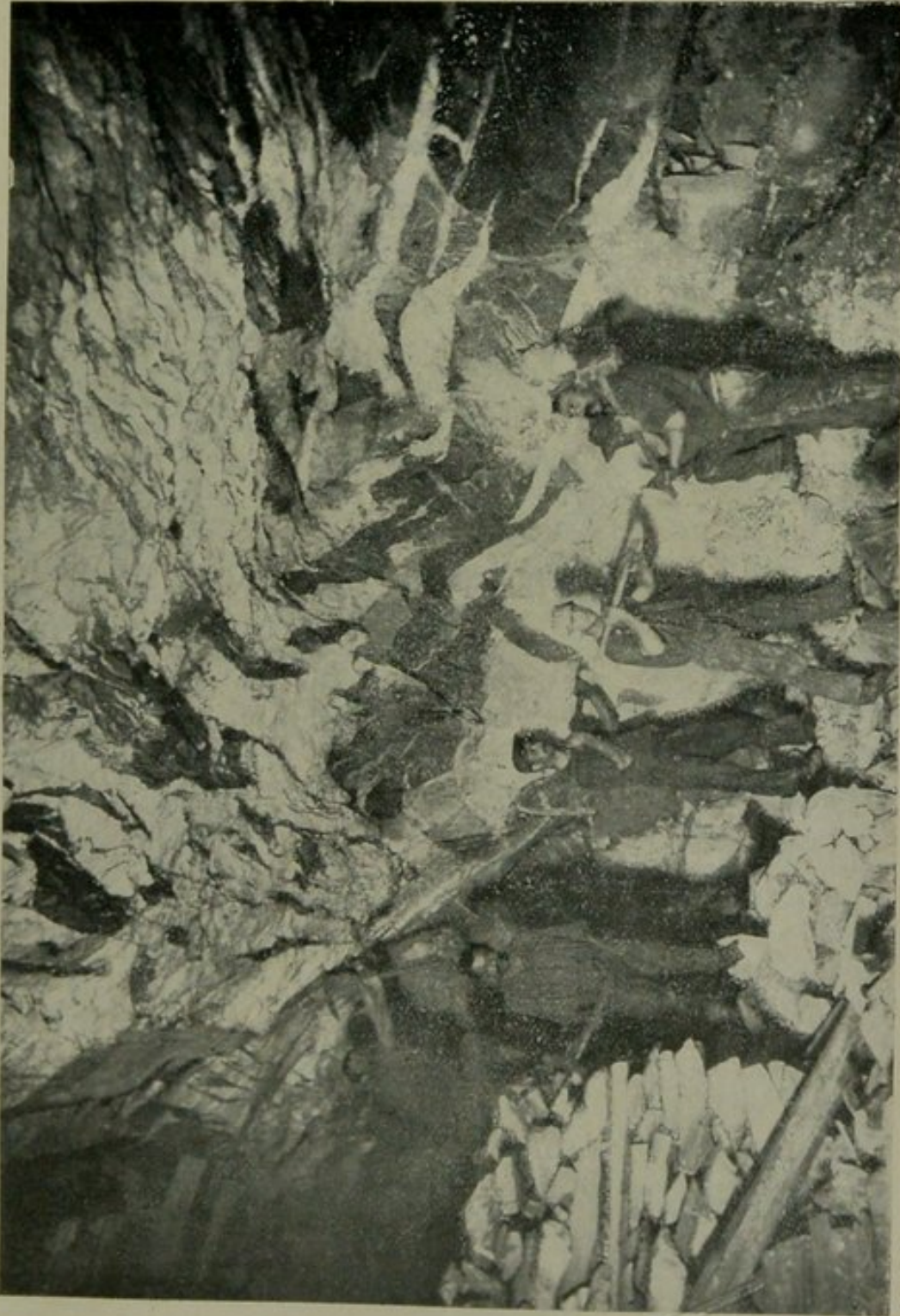
MASSIVE SPUR (IRREGULAR FORMATION) ON THE CATHERINE REEF, WORKED BY STOPPING. Photo. by W. H. Robinson, Bendigo.
