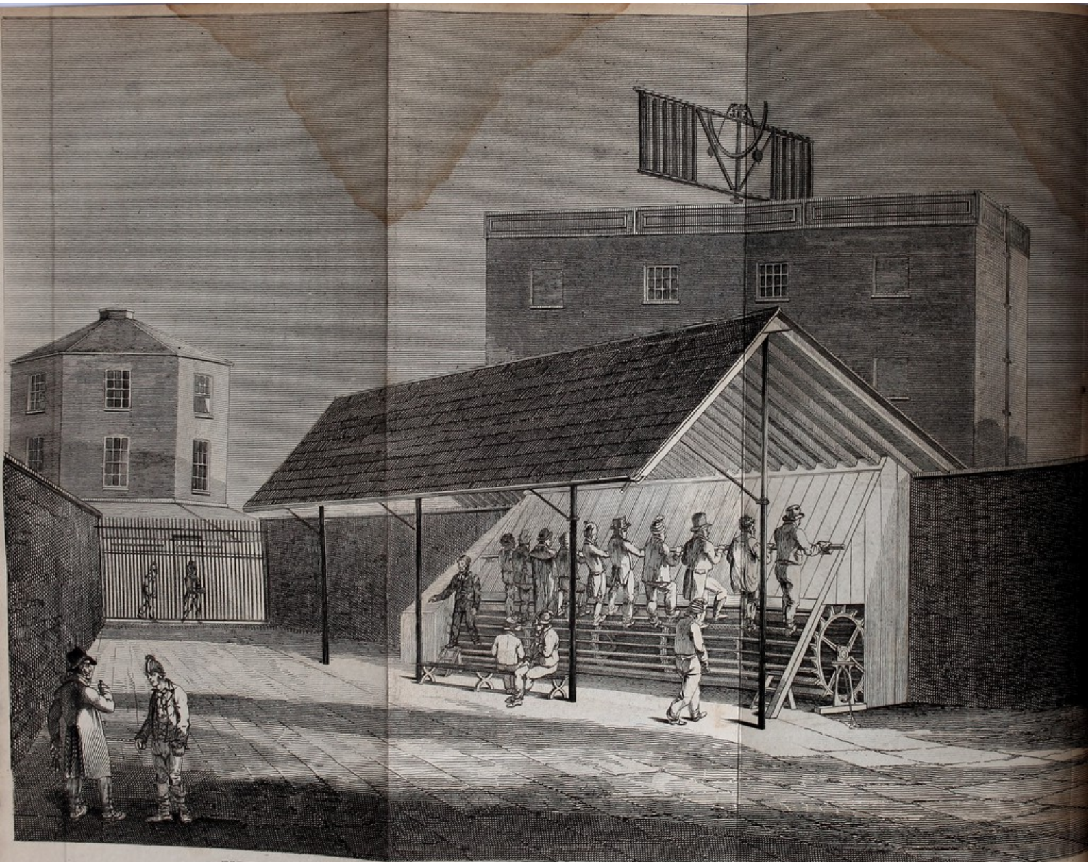
VIEW OF THE TREAD MILL FOR THE EMPLOYMENT OF PRISONERS, ERECTED AT THE HOUSE OF CORRECTION AT BRIXTON, BY M r W m CUBITT OF IPSWICH.
