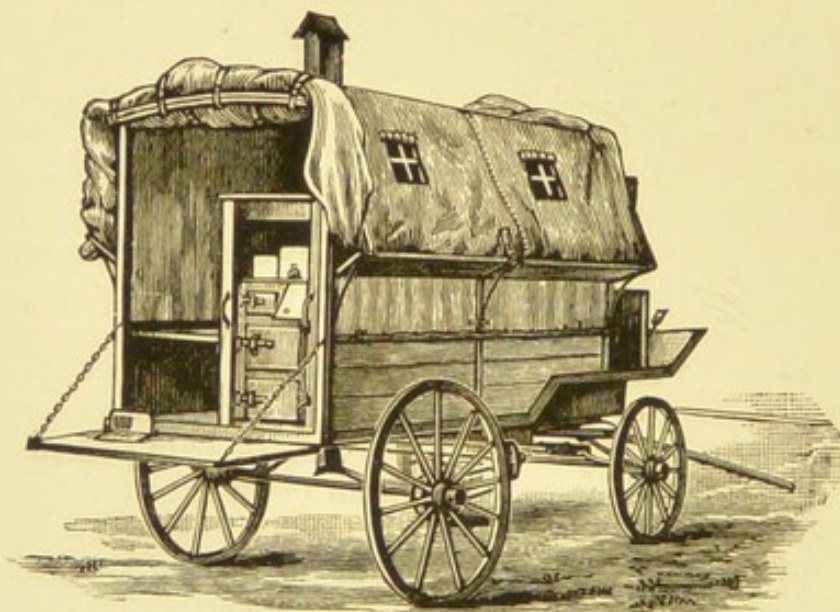
Fig. 144.—"Tortoise" waggon with "tortoise" tent folded. As a rule the waggon is made to act as a central support for the tent.
