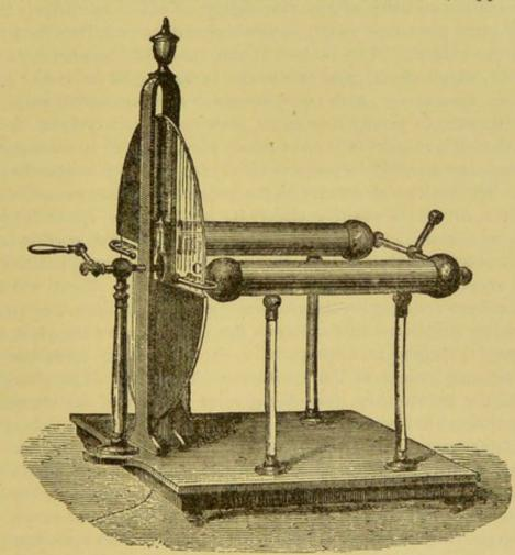
FIG. 1.-ONE FORM OF PLATE-GLASS MACHINE (THE RUMSDEN).
