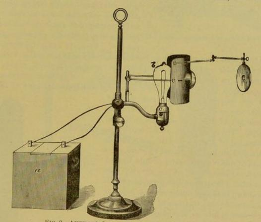
FIG. 2.-AUTHOR'S LAMP FOR ELECTRIC ILLUMINATION. a, storage battery; b, incandescent lamp; c, circuit closer.
