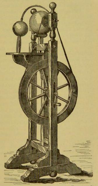
FIG. 8.—ENGRAVING OF BENJAMIN FRANKLIN'S ELECTRICAL MACHINE, THE OLDEST IMPROVED FORM FOR PRODUCING ELECTRICITY FOR EX-PERIMENTAL PURPOSES.
