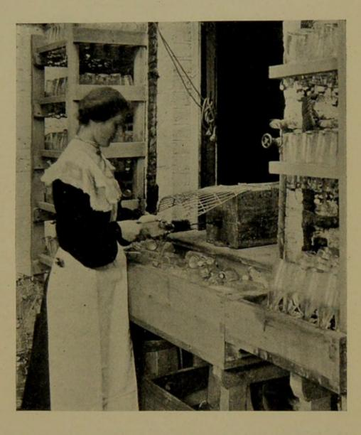
INFANTS MILK DEPOT, BATTERSEA.—BOTTLE-WASHING. The bottle is placed on a revolving brush driven by an electric motor.
