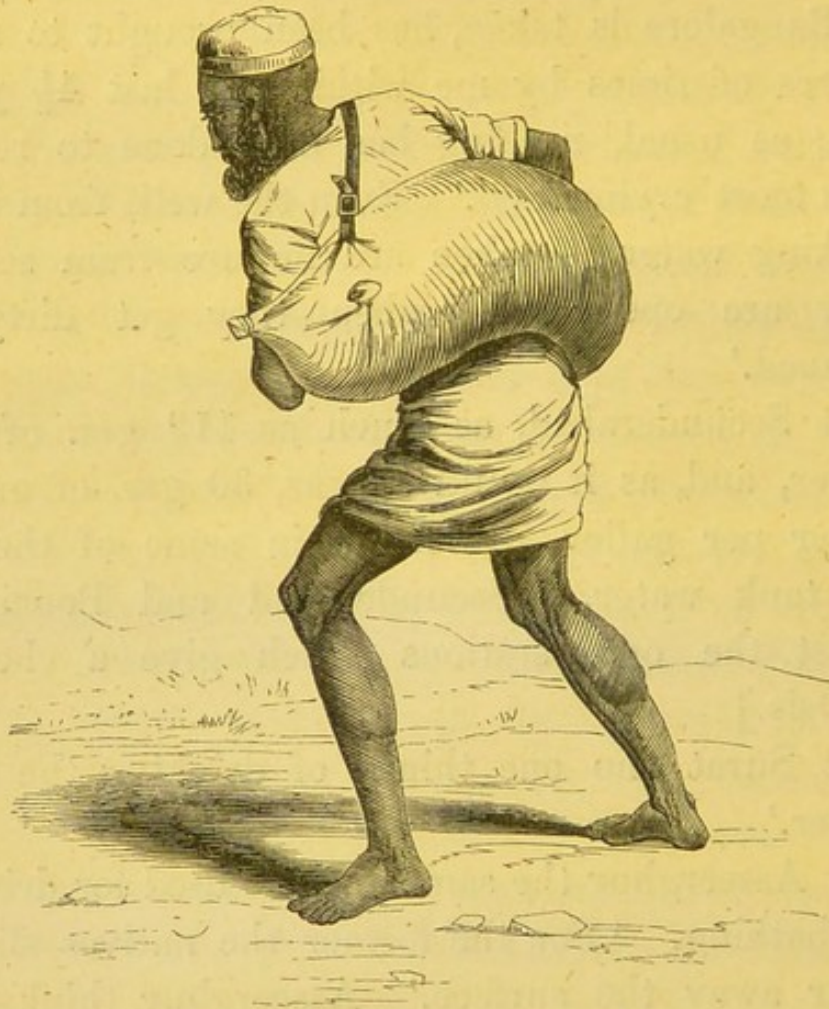
BEGINNING OF WATER PIPE.*
