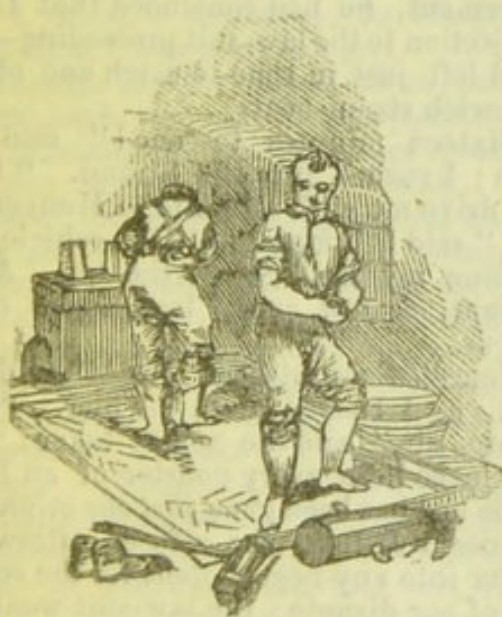
TREADING CLAY FOR STEEL CASTING POTS.
