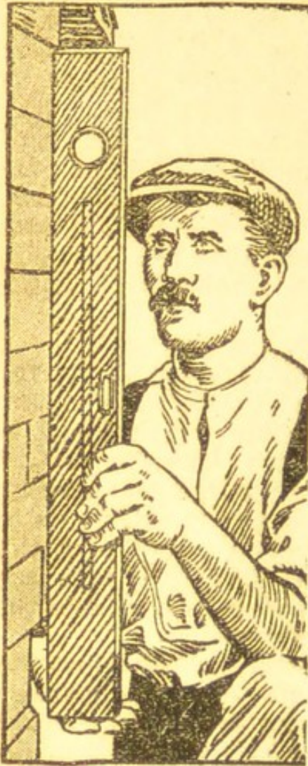
SPIRIT LEVEL. Testing an upright
