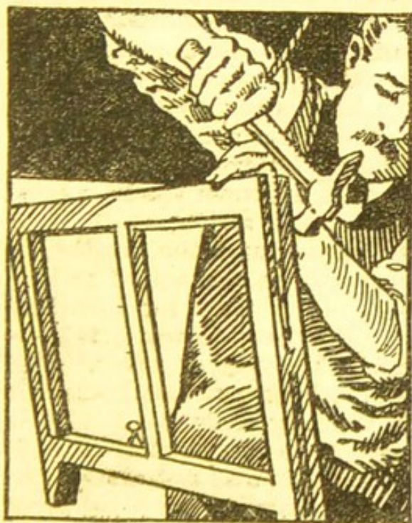
SASH. Fig. 4. Fixing new cord to sash with nails
