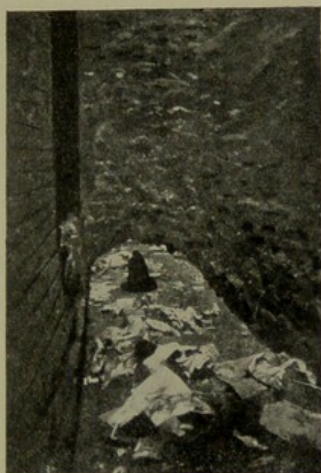
FIG. 104.—The bottom of an old-law air-shaft.
