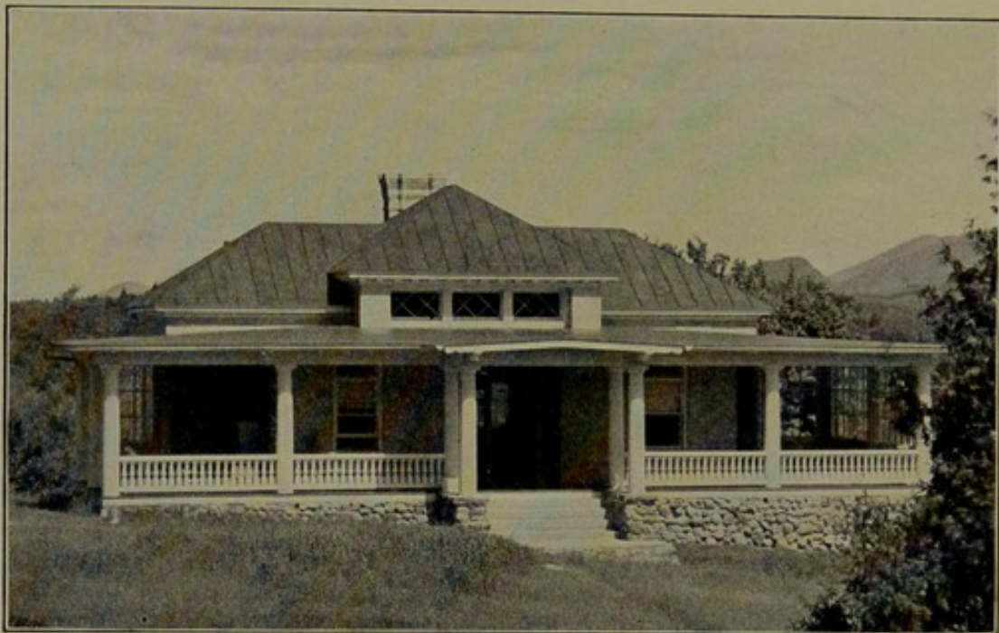
FIG. 56—Nathan cottage, Adirondack Cottage Sanatorium.
