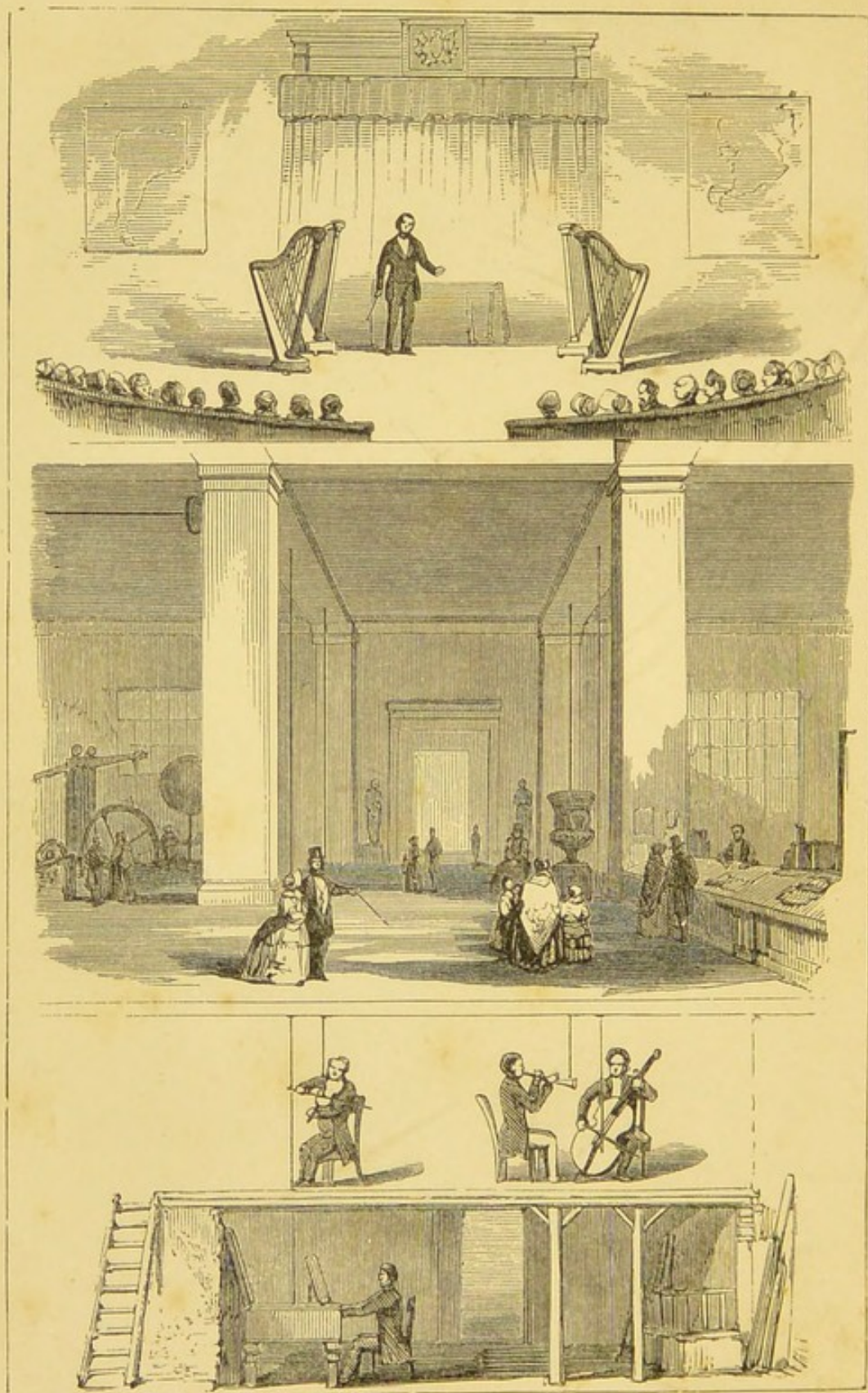
Wheatstone's telephonic concert at the Polytechnic, in which the sounds and vibrations pass inaudible through an intermediate hall, and are reproduced in the lecture-room unchanged in their qualities and intensities.
