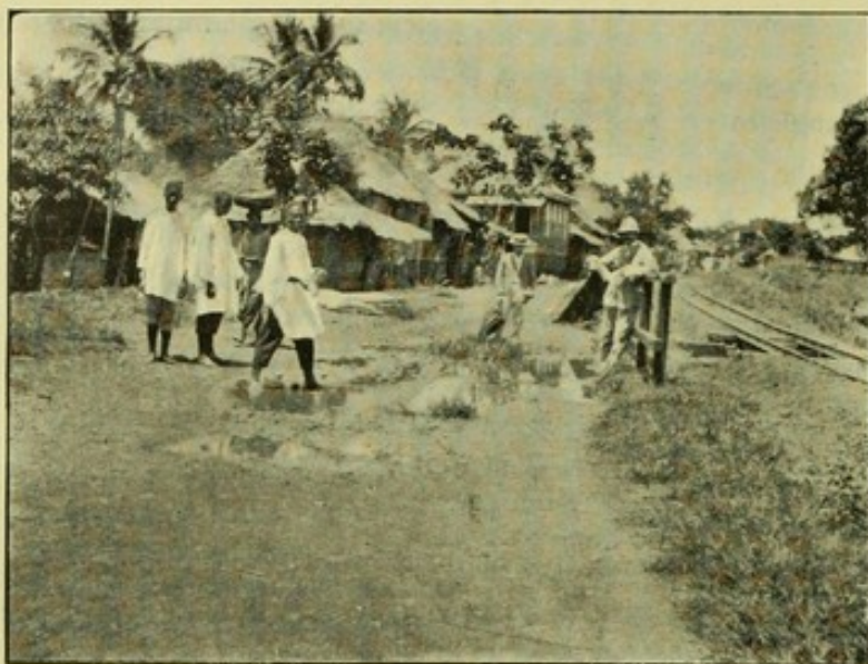
5. Large Anopheles pool produced by railway embankment.
