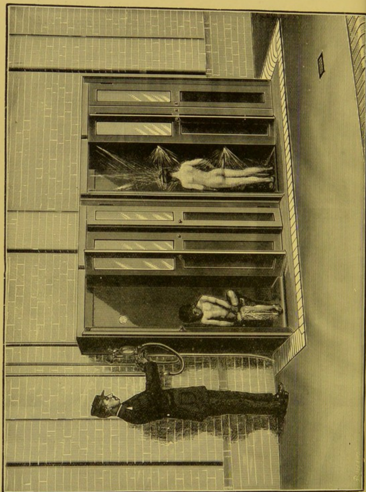
FIG. 24.—Spray baths used at the Strand Schools. The lad in the right hand compartment is having a body douche, while the one in the other compartment is washing his feet at an ascending spray.
