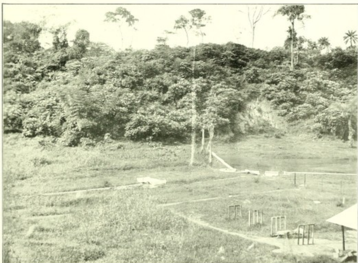
Calabar water supply, showing how spring can be contaminated by surface drainage.
