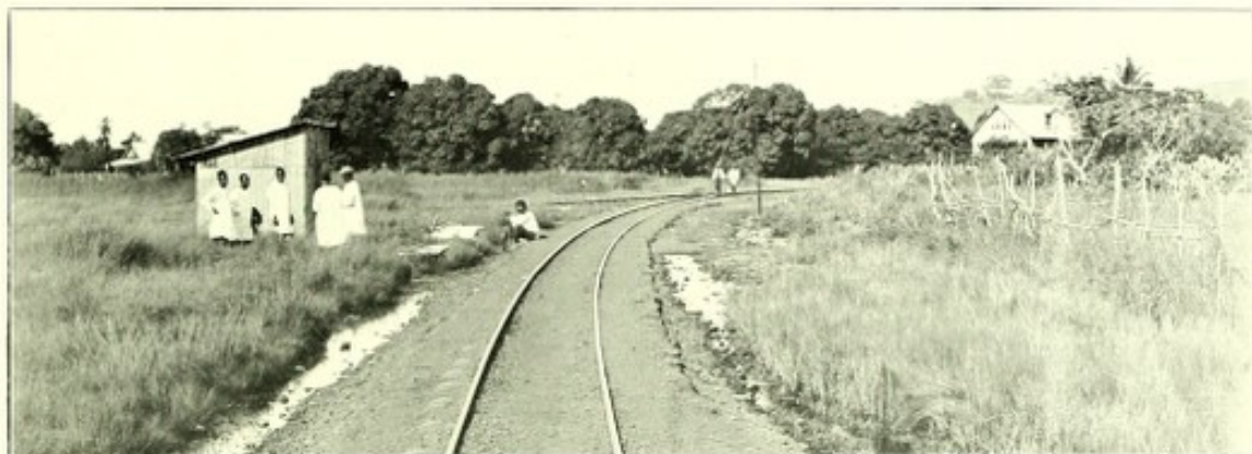
Grass fields near golf course, showing stagnant drains on each side of railway.
