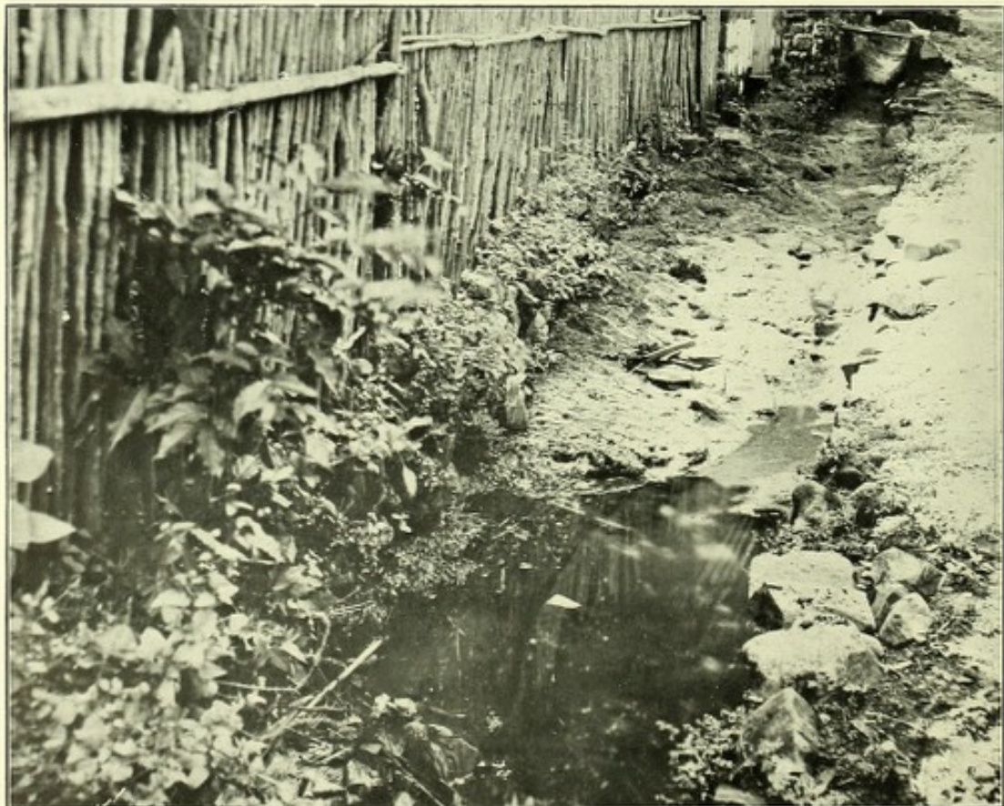
Rough rock drain—rock holes—drain dry above—spring lower down, making pool. [See page 26.
