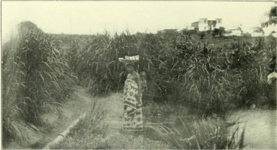
Essikadà main drain forming pool. Native-made footpath crosses it here. Woman standing in the pool. European hospitals to right on hill. Pipe at left base from a well for the railway yard water tank. The rank vegetation favourable to mosquitoes and tsetse fly.
