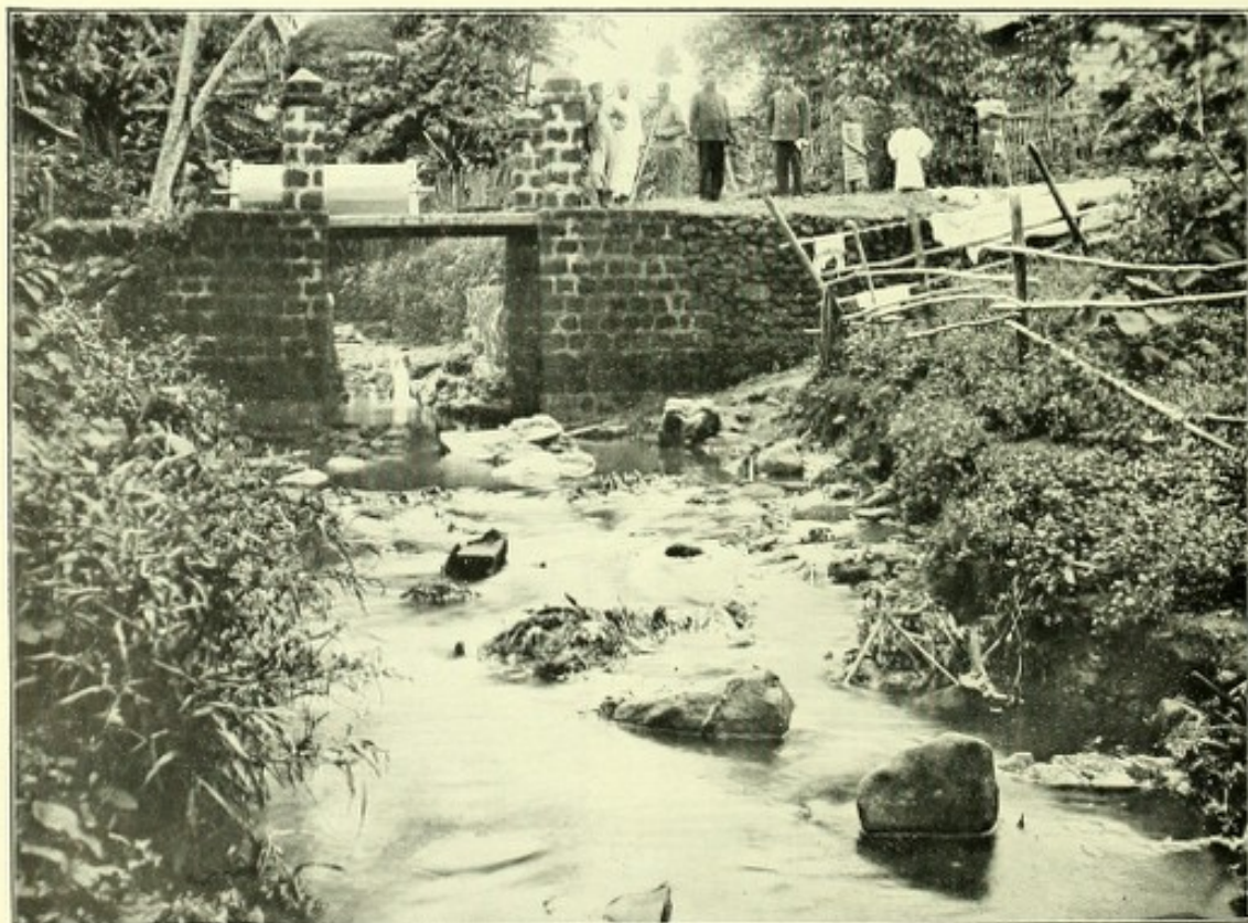
Nicol's Brook, showing canalization by rock cutting at further side of bridge. On near side bridge clothes washing and rubbish.
