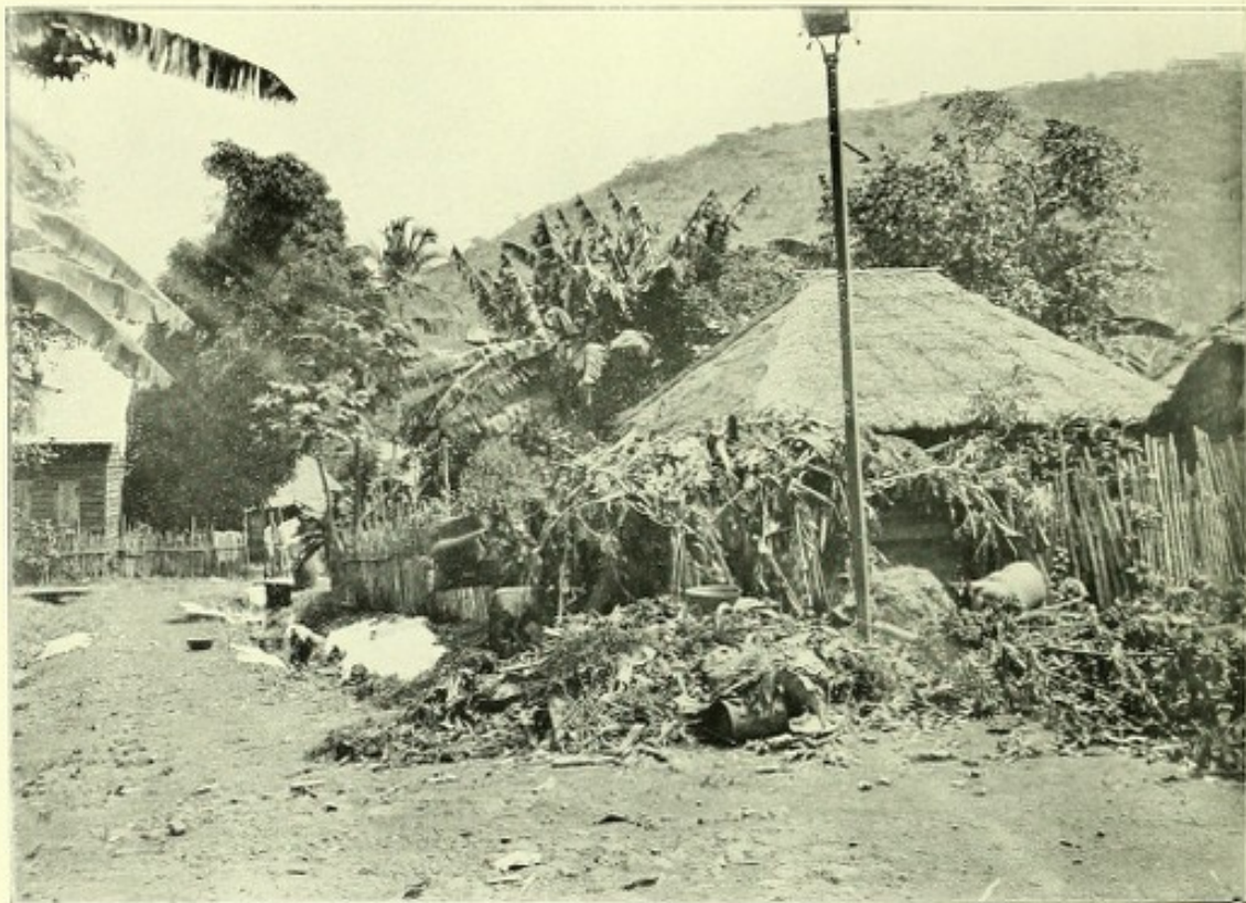
Overfilled rubbish bin—Circular road—washing in rough shut drain beyond.
