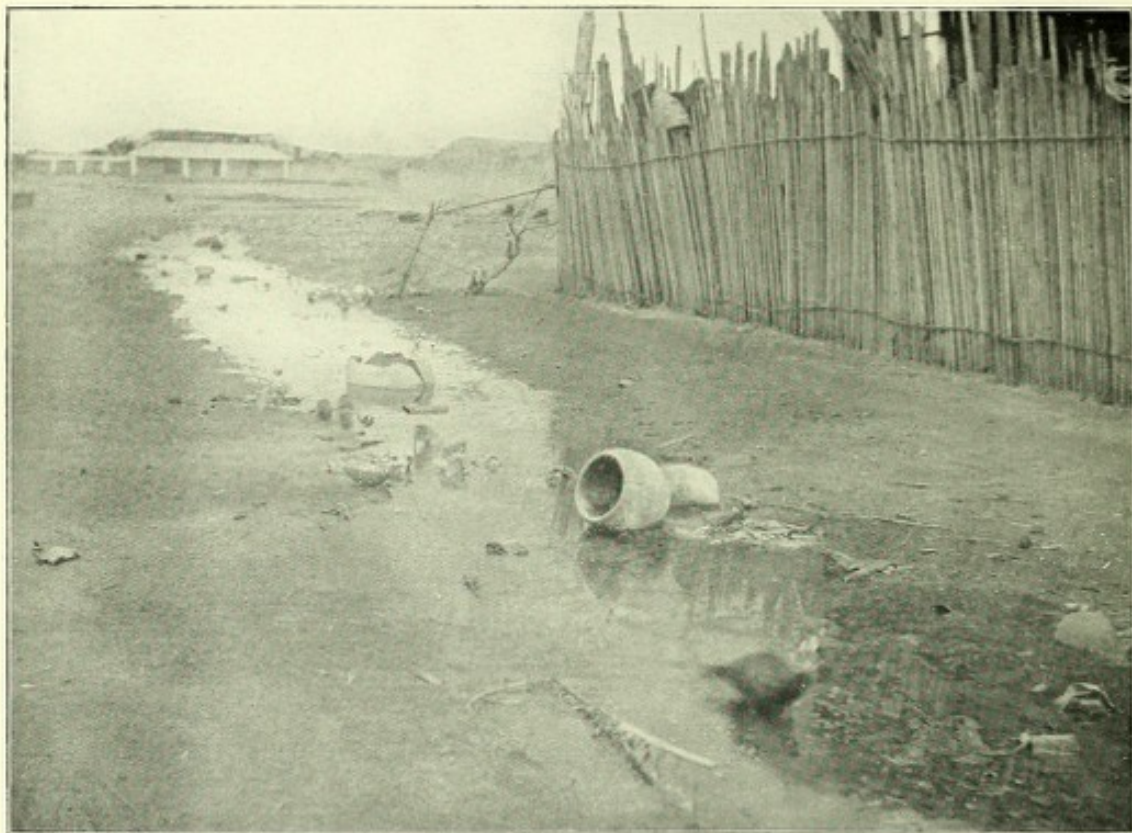
8 February, 1908. Alakoro reclamation. Kosh Street before reclamation.
