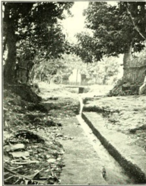
Rock-cut channel in bed of Sanders Brook in dry season with irregularities in surface on both sides.
