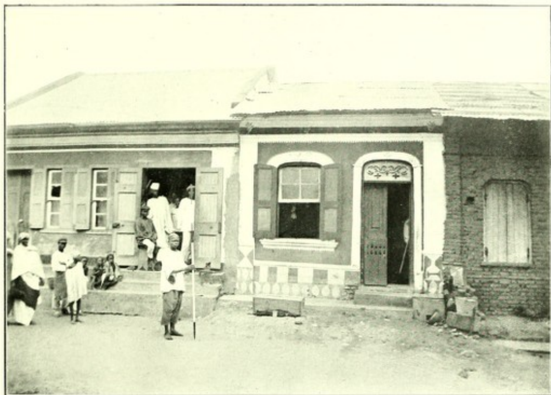
Badly planned house showing good frontage.
