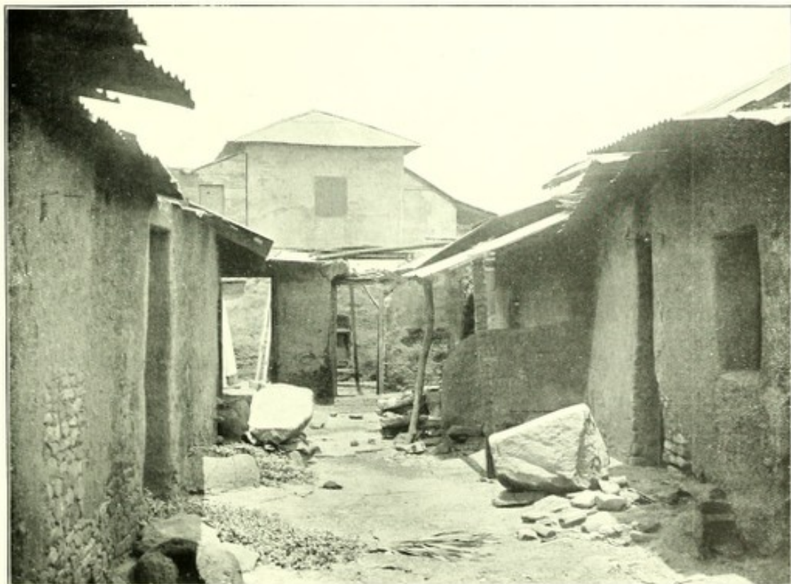
Condition of a courtyard common to two ranges of badly ventilated and badly lighted huts. No drainage, yard with many puddles during the rains.
