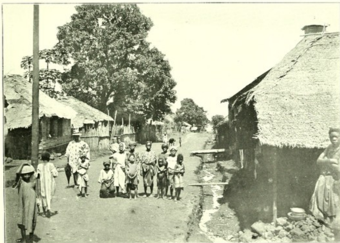
Little Kroo Street. Stagnant drain.
