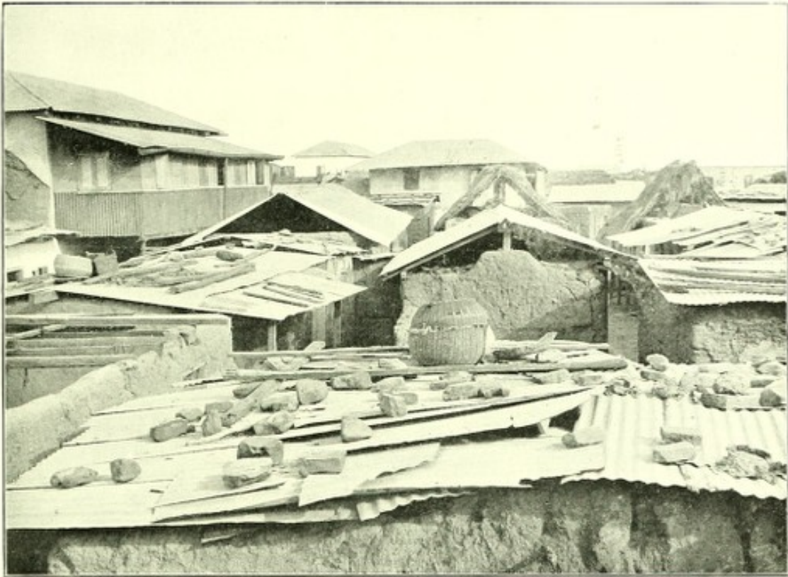
An insanitary area, showing huts and houses crowded together without roadways or good compounds. Nothing but demolition of the huts and remodelling the whole area can render it healthy.
