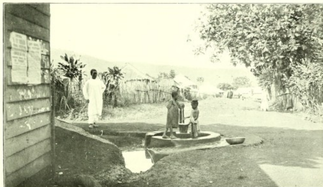
Stand-pipe, Circular road, showing pool chiefly from waste water, gravel washings from left blocking culvert—the larger mound of gravel is material removed from culvert mouth.
