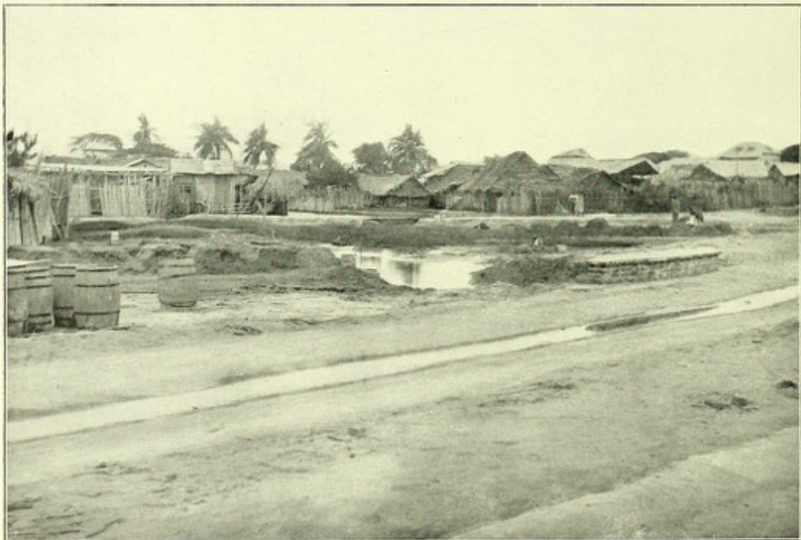
Alakoro Swamp, 13 July, 1908. Since filled in (12 Aug. 1908). In the foreground the formation for new road from Customs to Carter Bridge and new surface drains.
