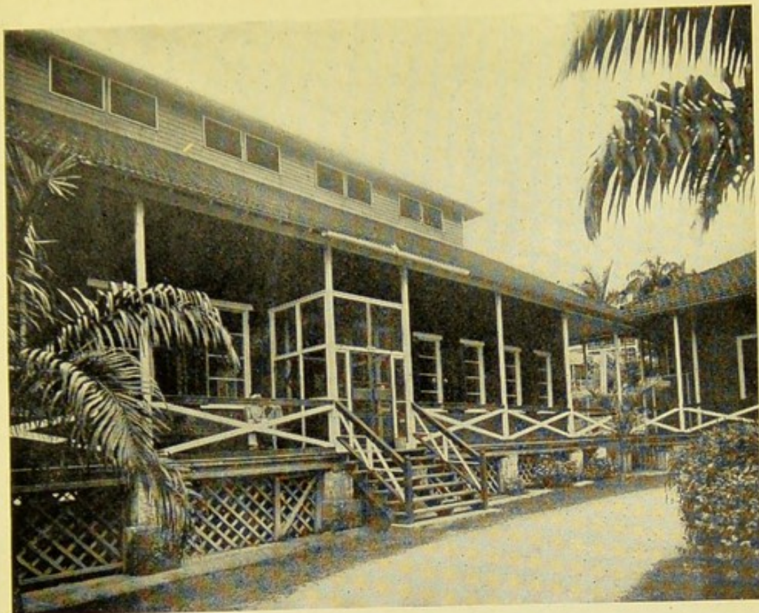
Screened Yellow-fever Ward. Ancon Hospital, Panama.
