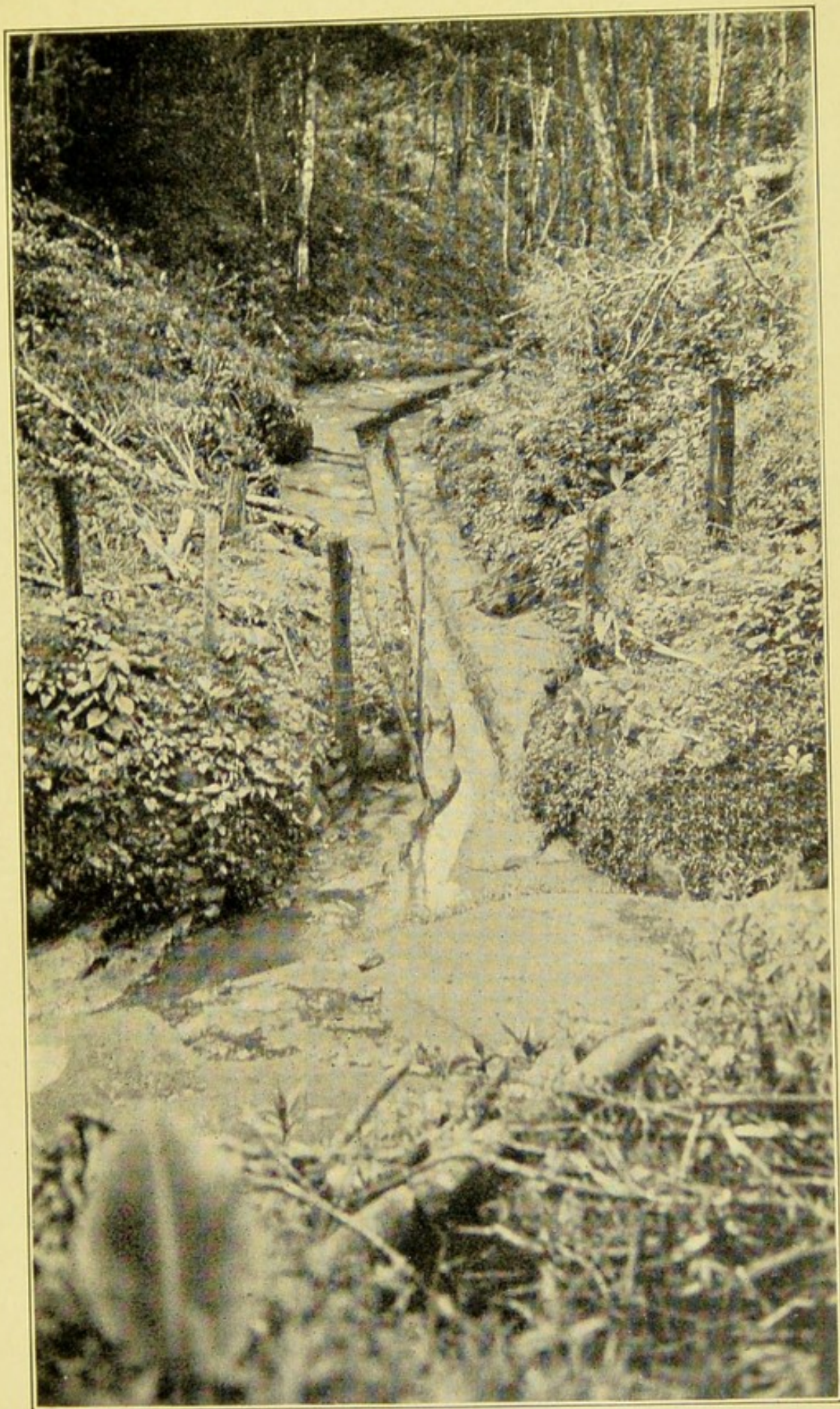
Concreted Ditch. Gatun.
