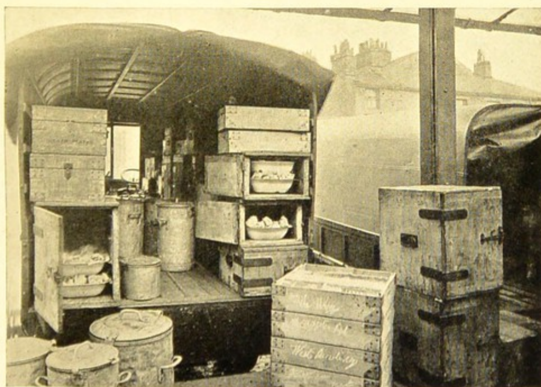
INTERIOR OF MOTOR WAGON. SHOWING DEVICES FOR RETAINING HEAT. BRADFORD, ENGLAND
