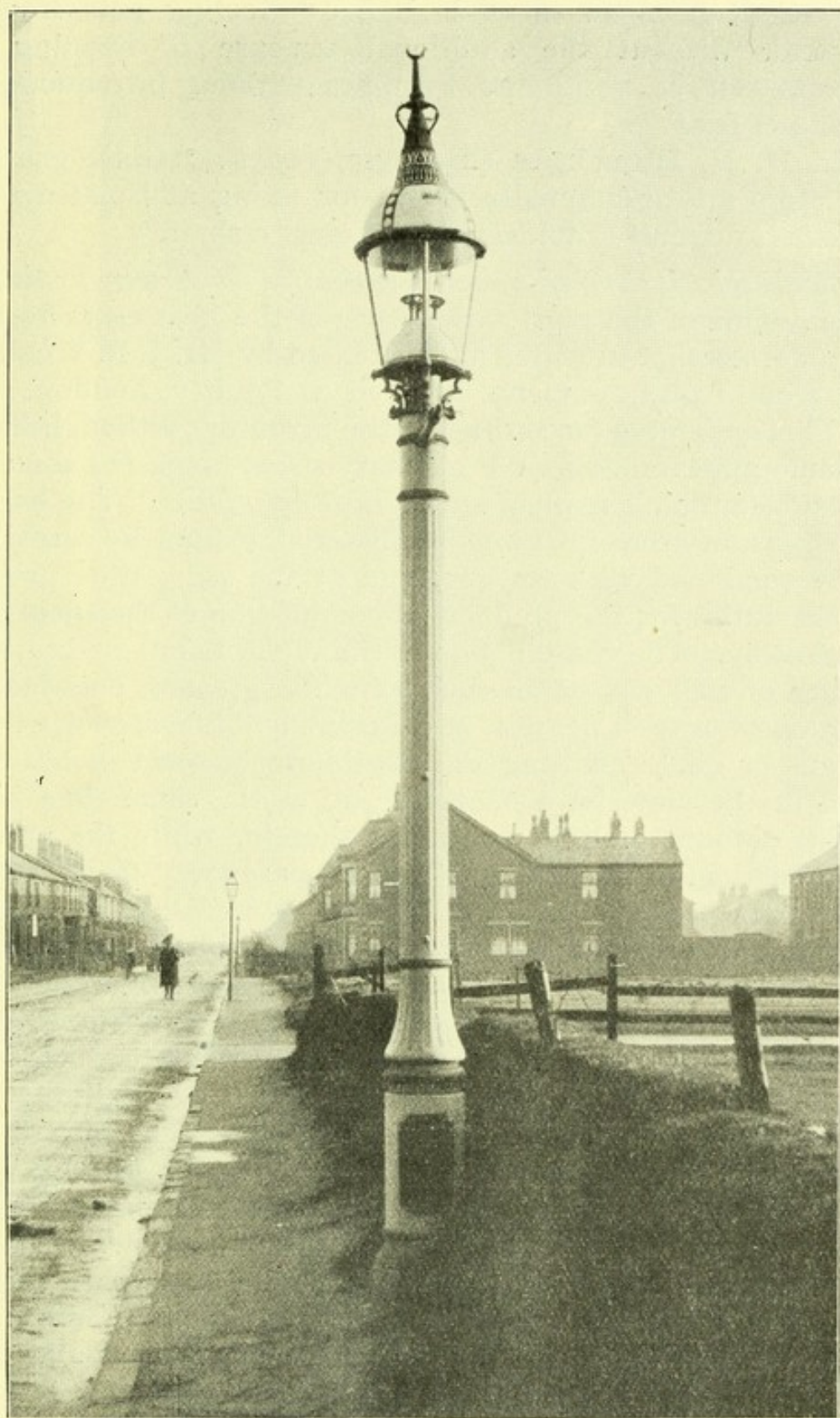
FIG. 9. WEBB'S SEWER VENTILATING LAMP AT BLACKPOOL.
