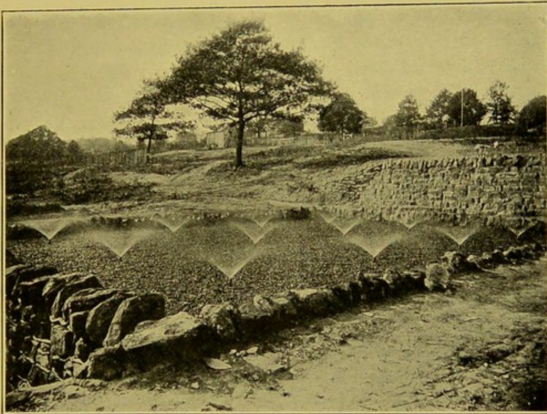
Fig. 49.—Fixed Sprinklers in Operation at Tunbridge Wells.
