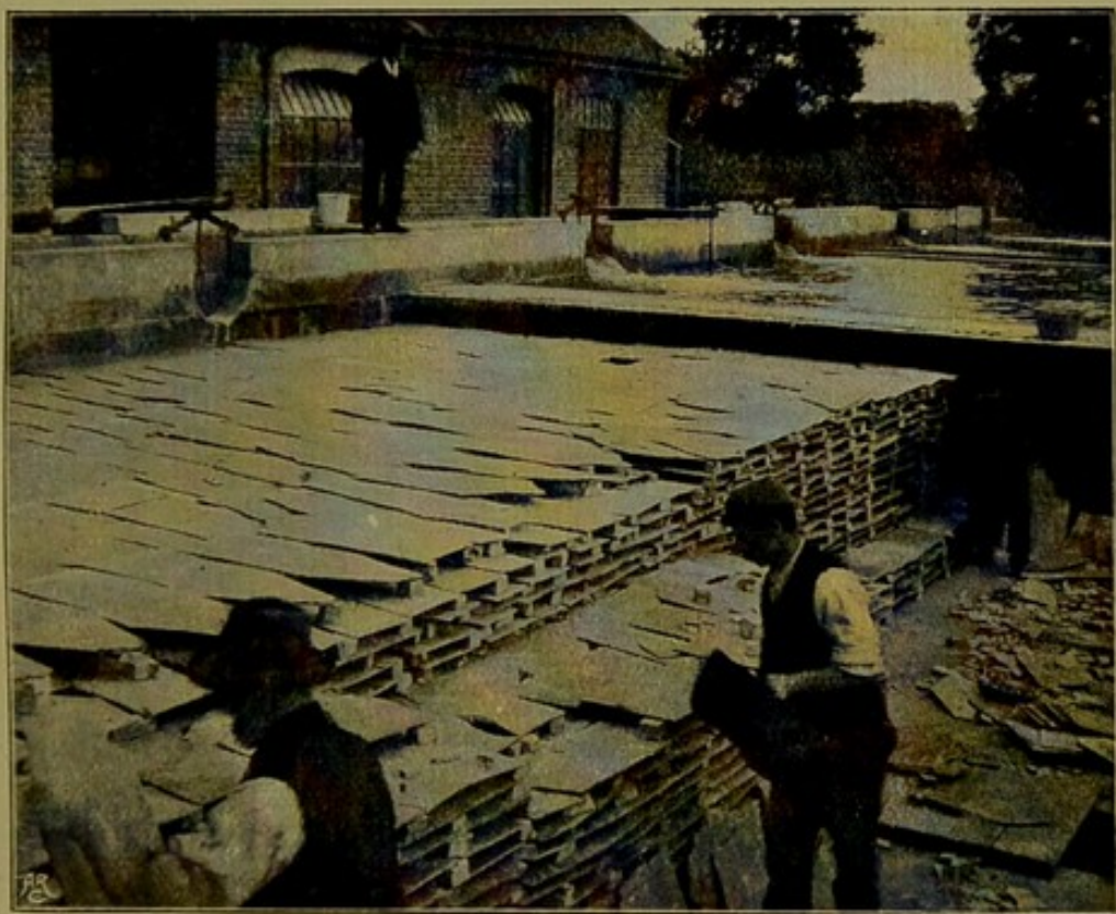
FIG. 8. FILLING THE SLATE BEDS AT MALDEN, SURREY.
