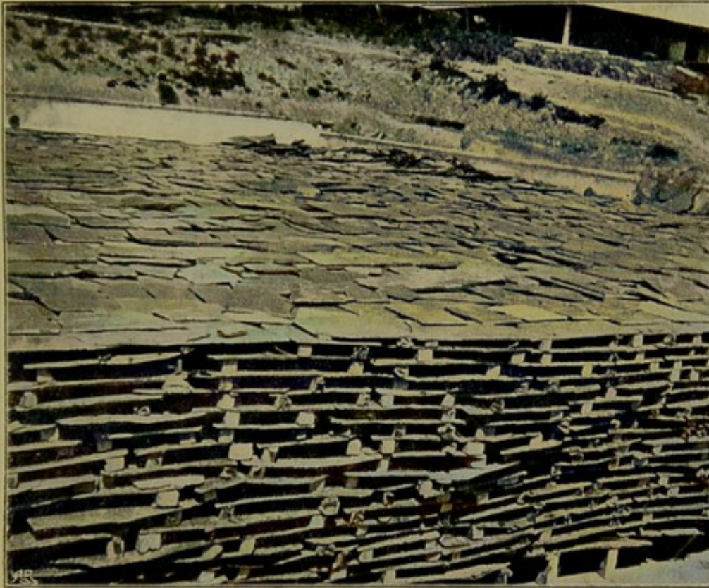
FIG. 6. DEVIZES PRIMARY BED. Section showing Slate Layers. (See Fig. 8.)
