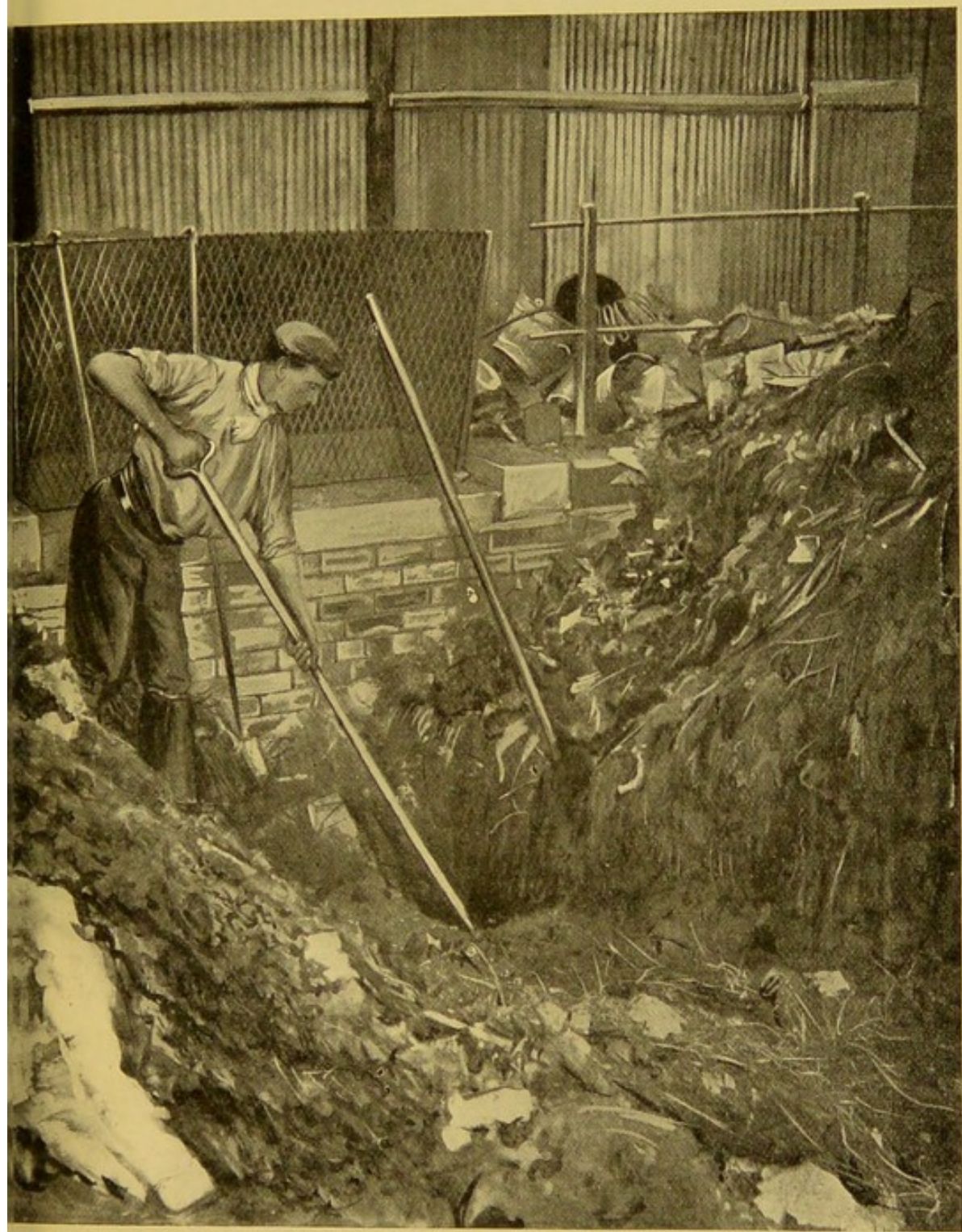
FIG. 58. BRADFORD (HAMMERTON STREET) DESTRUCTOR. View on top of Cells showing the Charging Operation.
