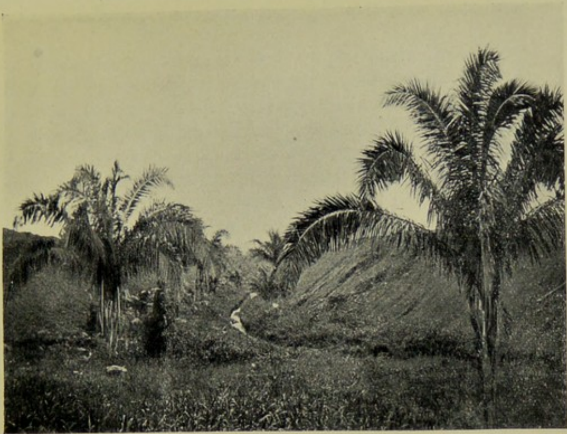
FIG. 29.—The photograph shows to what depth the swamp at Culebra has been filled.
