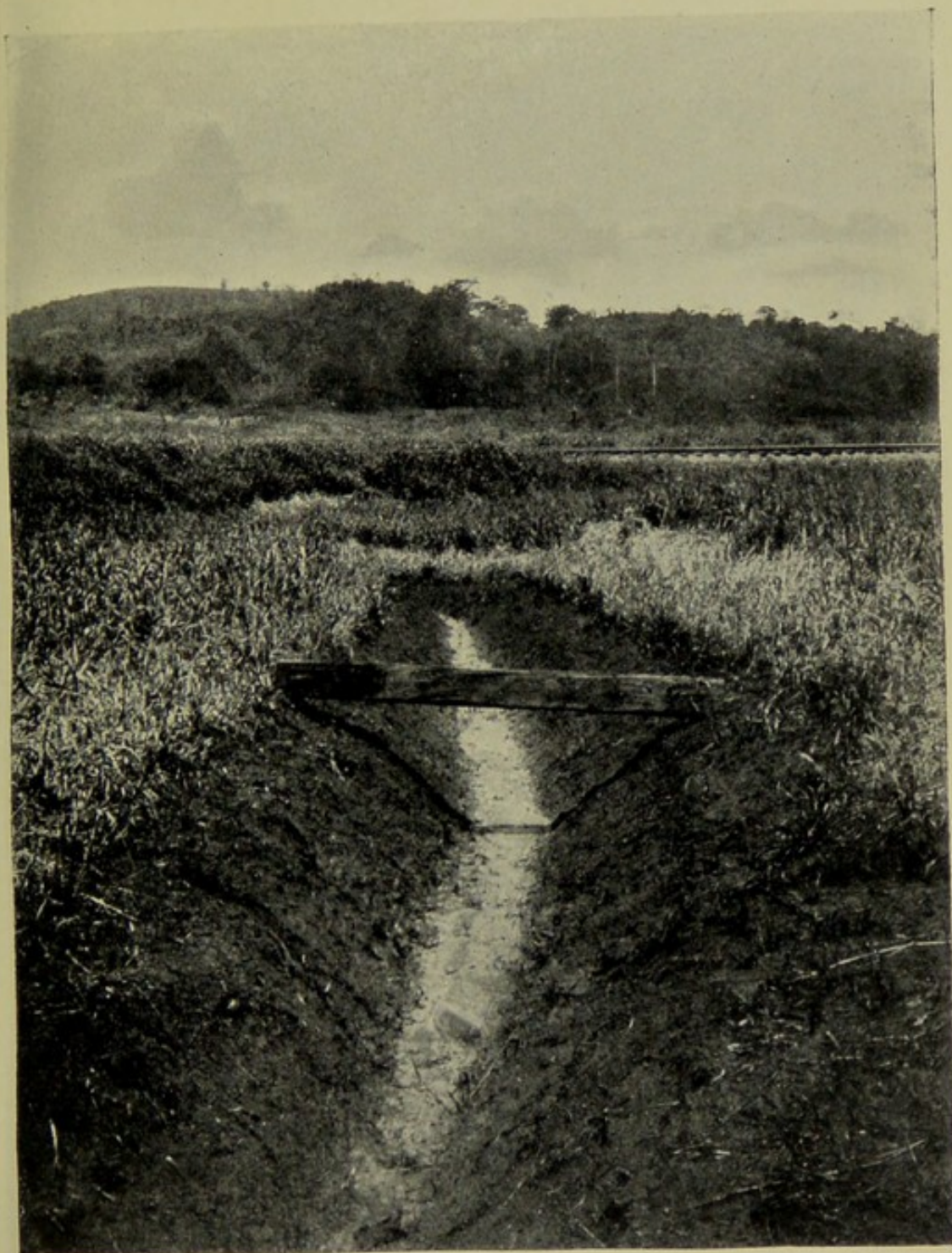
FIG. 21.—SHOWS A DITCH WHERE THE GRASS HAS BEEN CLEARED BY BURNING, MIRAFLORES STATION.
