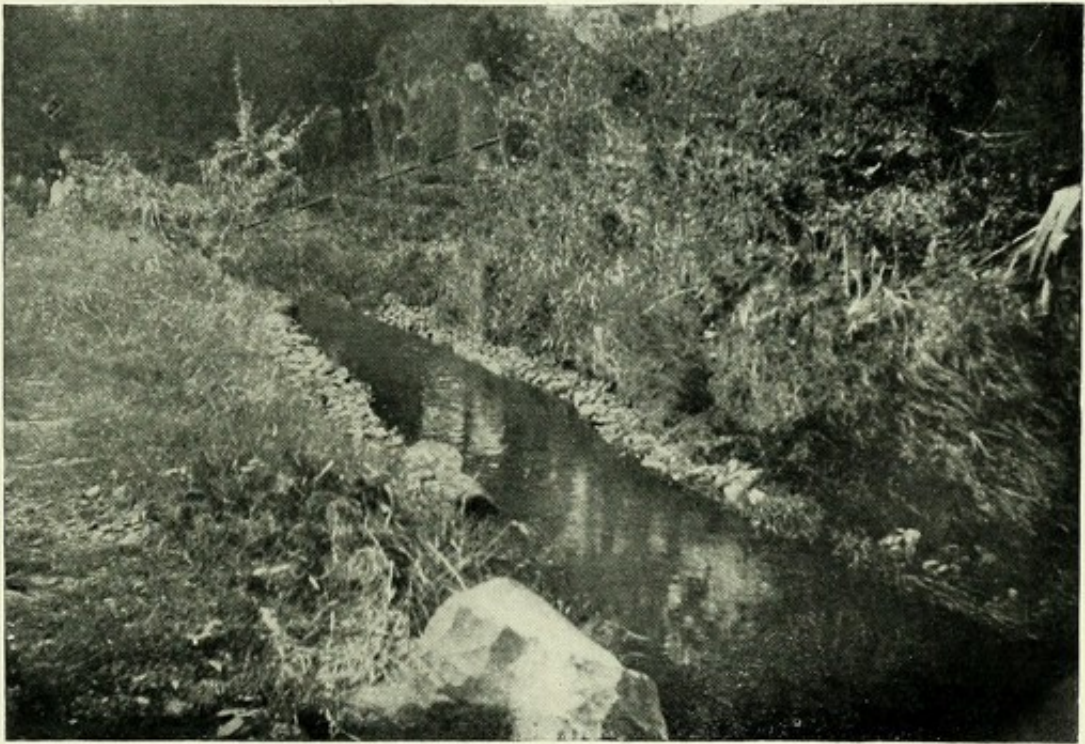
PHOTO. 24.—Rough canalisation of Latanier River, Port Louis.
