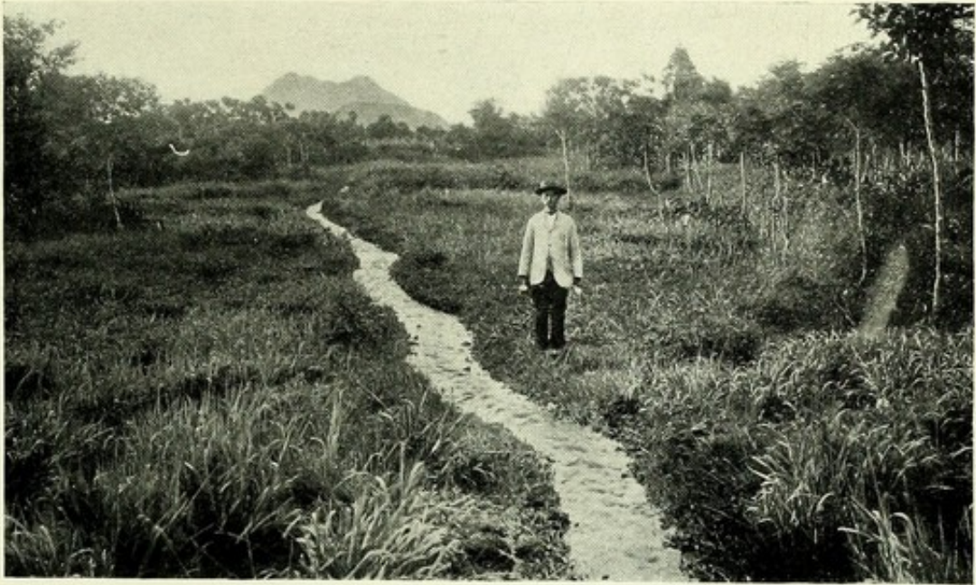
PHOTO. 23.—Part of channel at Clairfond Marsh cleared by three men in one day.
