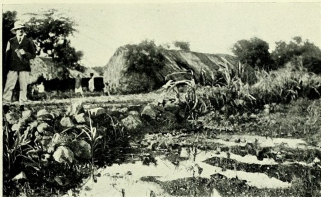
PHOTO. 13.—Marshy condition at Clairfond, made by a Conservancy Road.
