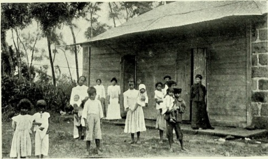
PHOTO. 7.—Middle-class Creole's House at La Caverne.
