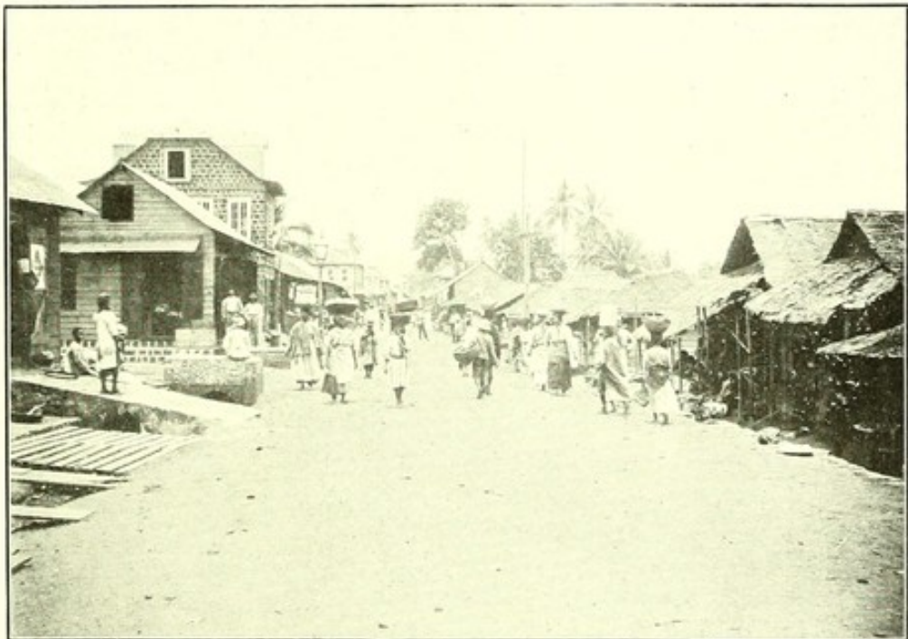
A STREET IN FREETOWN, SHOWING DRAIN AT SIDE AND NUMEROUS GANGWAYS OVER IT. HOUSES ON RIGHT SIDE ARE LOWER THAN STREET LEVEL.
