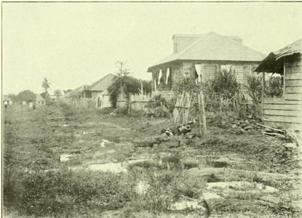
ANOTHER ROCK-POOL STREET SHOWING GROWTH OF WEEDS AND IRREGULAR HOUSES
