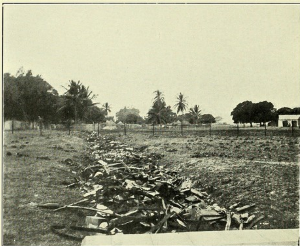
Preliminary filling in of a grass-clogged ditch at Bathurst with old tins, scrap iron, etc., collected from compounds in the town, the source of many mosquitoes, chiefly of the Anopheles genus.
