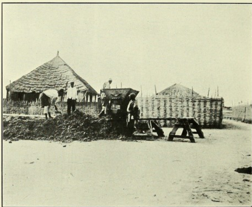
Raising the level of Halt Die Swamp by deposition of sand taken from the beach.
