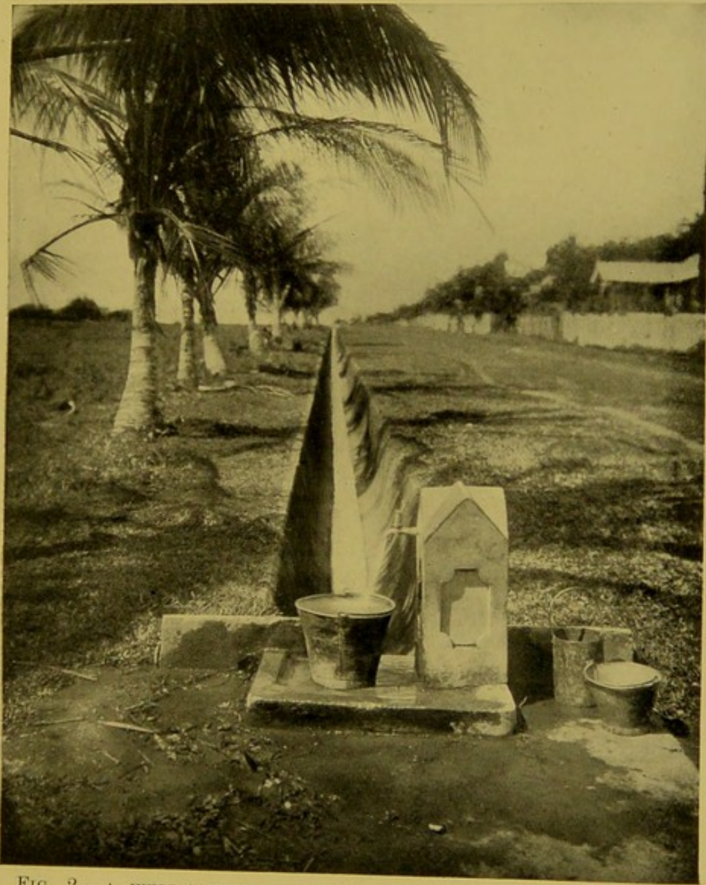
FIG. 2.—A WELL-CONSTRUCTED DRAIN AND STANDPIPE, THE AGENTS WHICH HAVE CAUSED THE DIMINUTION OF MOSQUITOS, TRINIDAD. p. 12]
