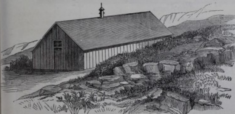
Hut with the Site excavated, and earth against the sides.
