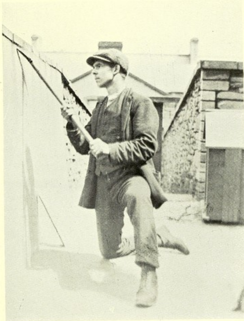
FIG. 23.—COLLIER CLEANING THE TOP OR TOP HOLING.
