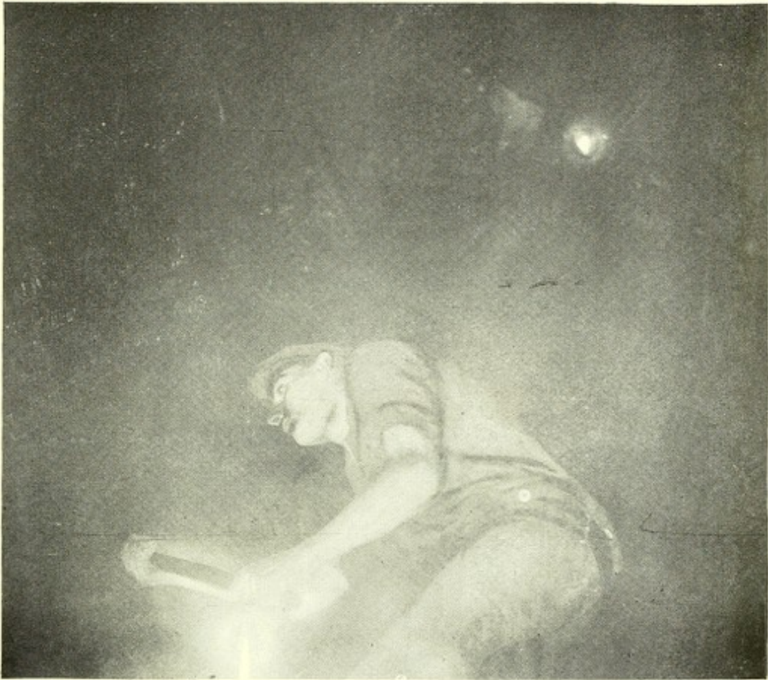
FIG. 15.—PHOTOGRAPH OF A COLLIER HOLING IN THE BOTTOM OF THE COAL.
