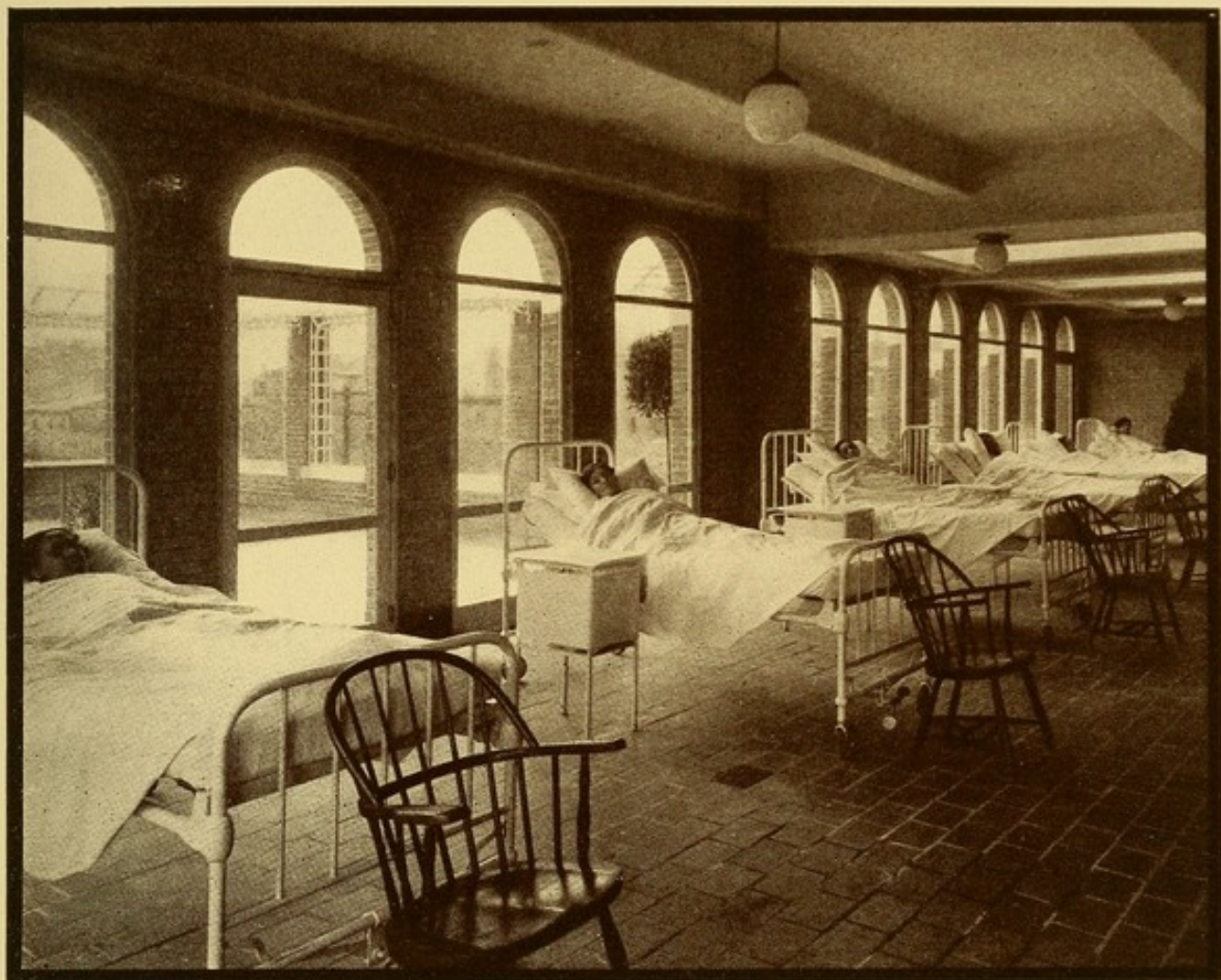
PORCH AND OPEN DECK ADJOIN- ING WARDS FOR ADVANCED CASES ON THE THIRD FLOOR
