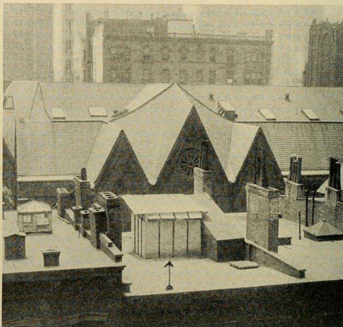
No. 16.—View of a shelter constructed of sheet iron nailed to a wooden frame on the roof of a brick building.
