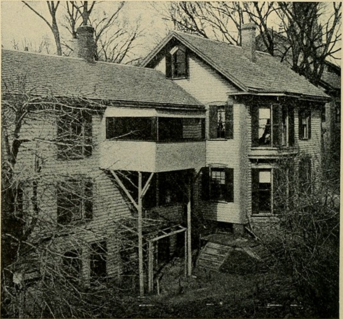
No. 36.—A temporary wooden porch placed for protection in an angle of the house and supported on four by four inch timber posts.
