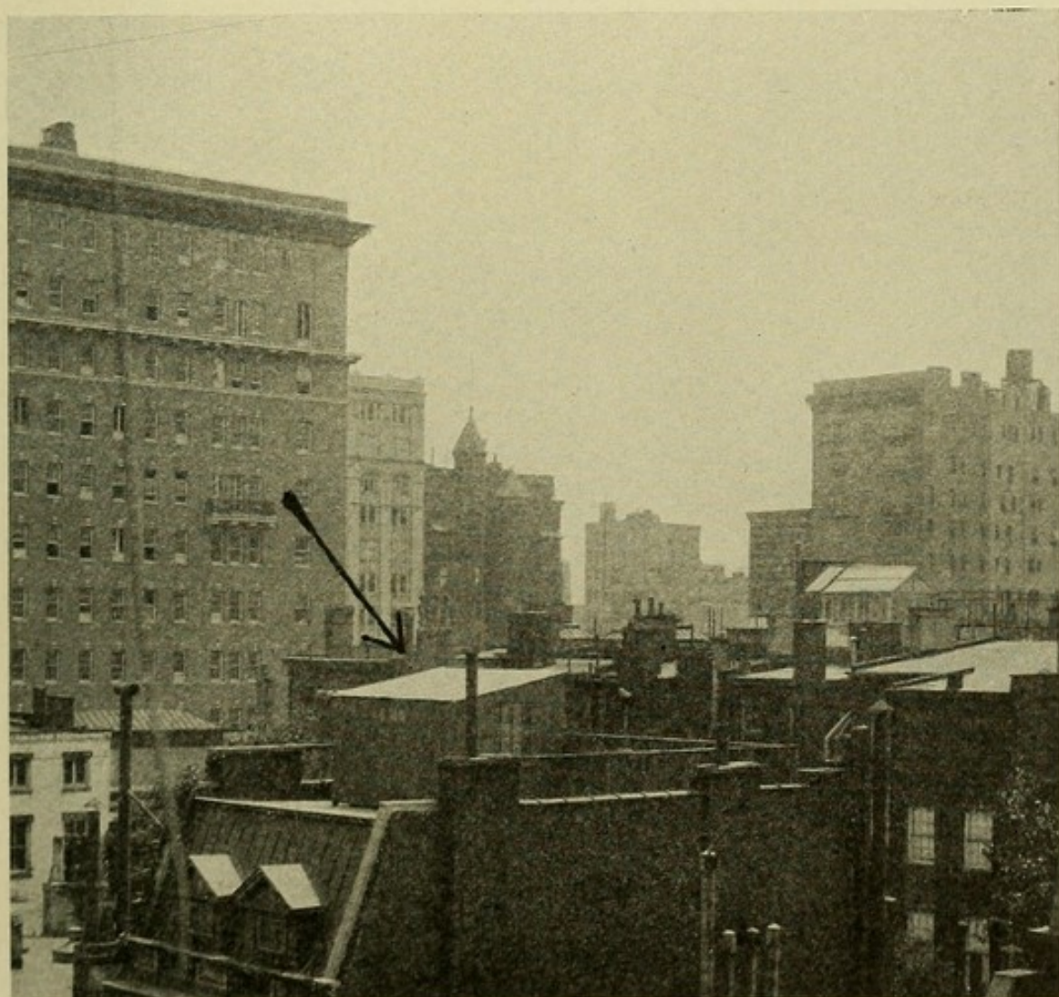
No. 17.—View of a shelter constructed of corrugated iron nailed to a wooden frame on the roof of a brick building.
