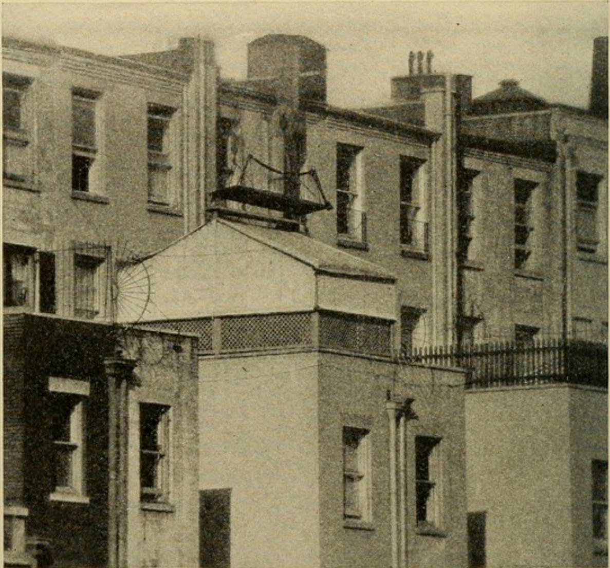
No. 65.—A tent on the roof of the rear extension of a city dwelling, raised over a rigid and well anchored frame. The lattice work base protects the interior but allows fresh air to enter. ( Courtesy of Dr. W. P. Northrup. )
