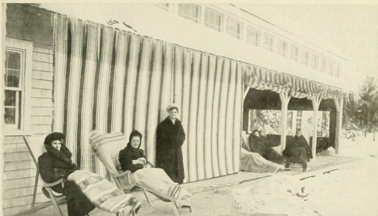
No. 70.—North Reading State Sanatorium, North Reading, Mass. JOHN A. FOX, ARCHITECT. VIEW OF AN OPEN PORCH, ILLUSTRATING A METHOD OF PROTECTING PORCHES BY CANVAS CURTAINS IN STORMY WEATHER. (See illustration 87 for further description of this institution.)
