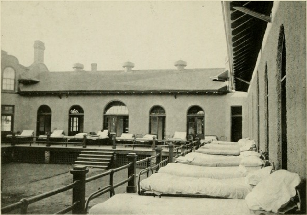
No. 55.—United States Army General Hospital, Fort Bayard, N. M. VIEW OF INNER COURT SHOWING SLEEPING PORCHES.
