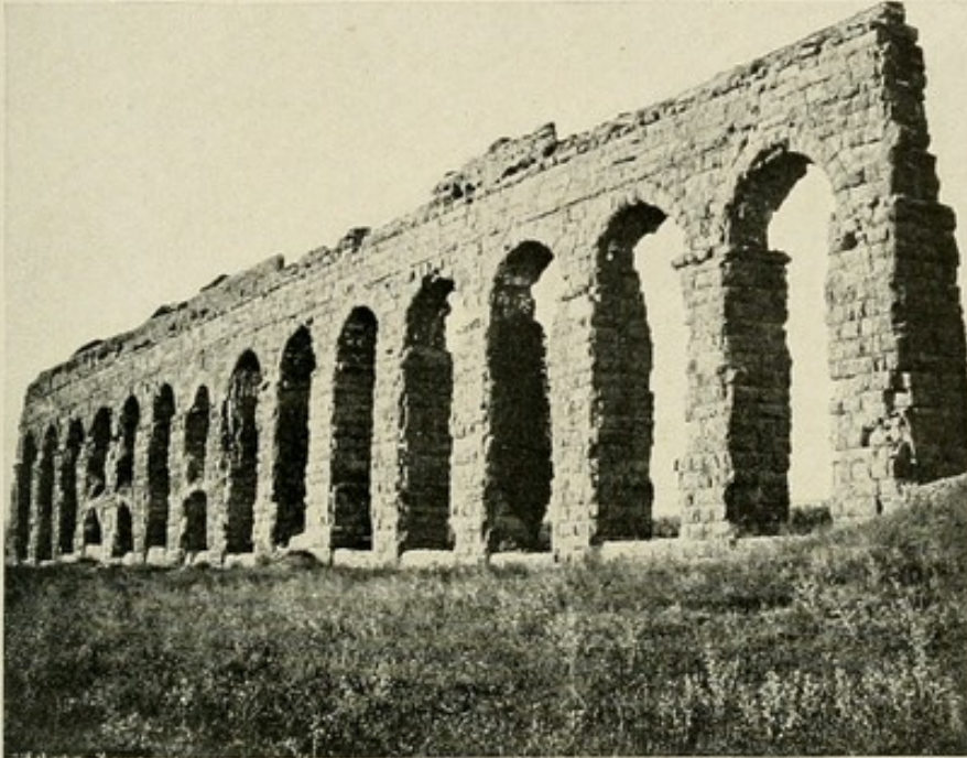
Near View of the Claudia Aqueduct
