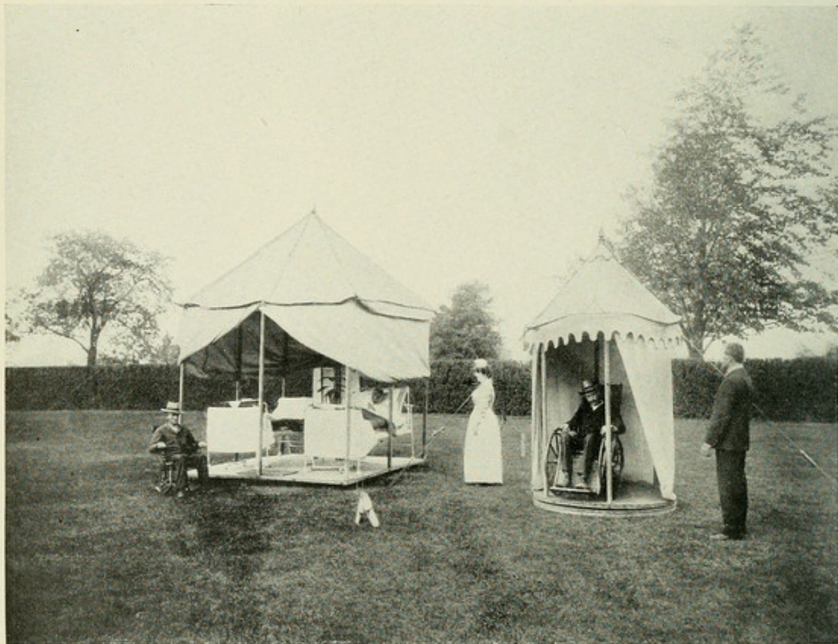
FIG. 2. MANHATTAN STATE HOSPITAL, EAST CAMP A. INSANE TUBERCULOUS PATIENTS. REVOLVING TENT CONSTRUCTED SO AS TO BE EASILY TURNED IN ACCORDANCE WITH THE DIRECTION OF SUN AND WIND.
