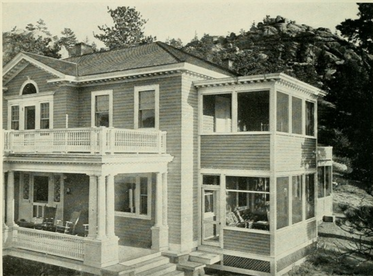
DOUBLE SLEEPING PORCH WITH EASTERN AND SOUTHERN EXPOSURES. THIS SUMMER RESIDENCE IN ESTES PARK, COLORADO, IS PROVIDED WITH PORCHES ON ALL SIDES SAVE THE NORTH, WHICH IS PROTECTED BY THE ROCKY FORMATION IN THE BACKGROUND. THE PORCH IS COVERED WITH A PERMANENT ROOF.
