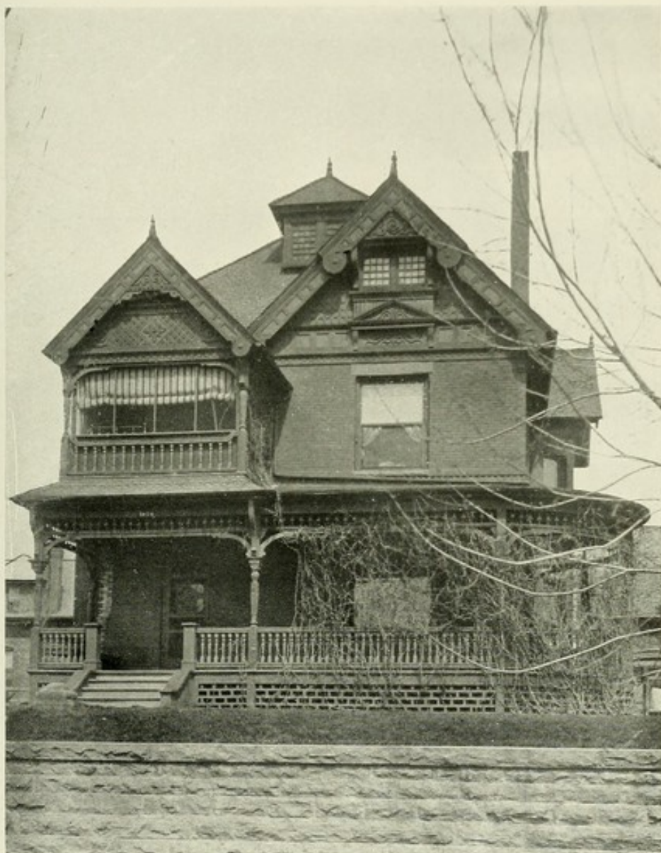
CITY RESIDENCE WITH IDEAL UPPER DOUBLE SLEEPING PORCH CONNECTED WITH BEDROOM. SHEATHING AT THE BASE, WIRE SCREENING, AWNINGS, ELECTRIC LIGHT.
