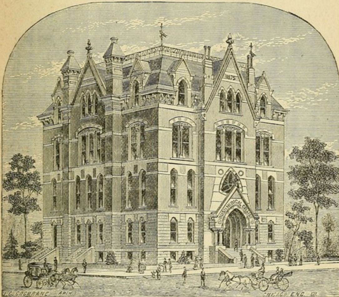
NEW EDIFICE OF RUSH MEDICAL COLLEGE NOW IN PROCESS OF ERECTION.
