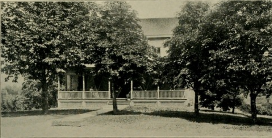
TEMPORARY RESIDENCE OF SUPERINTENDENT (CRAIG COLONY).
