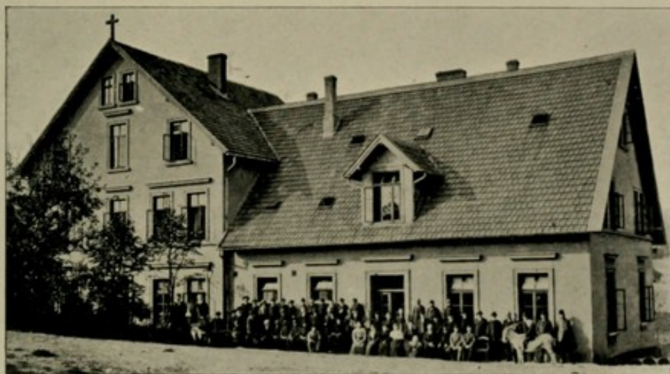
MAMRE — FARM RESIDENCE FOR EPILEPTICS.
