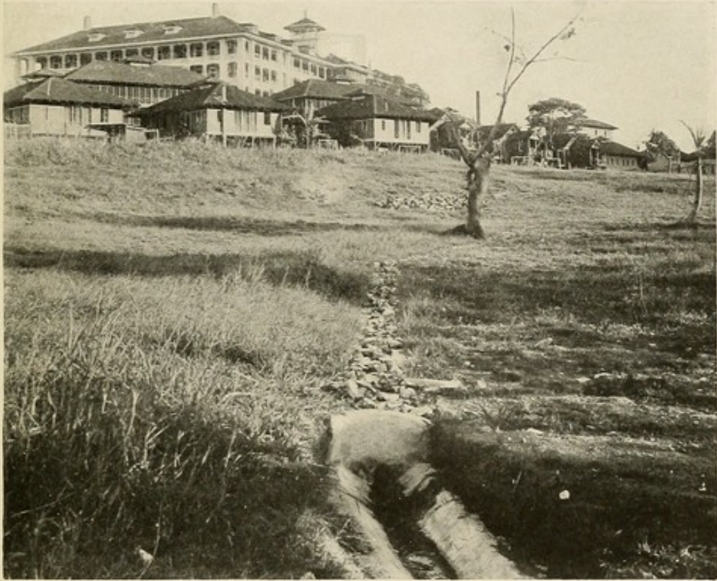
Oiled concrete drainage ditch near Ancon.
