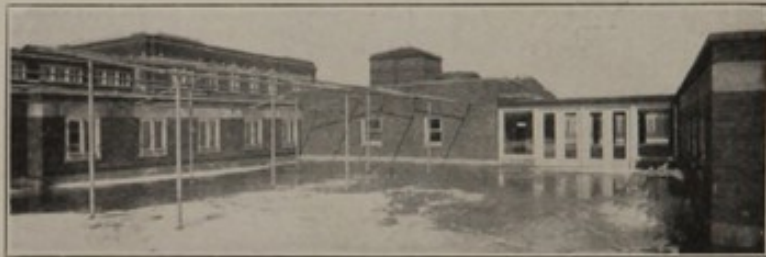
Fig. 11.—Roof garden—south end of ward A.
