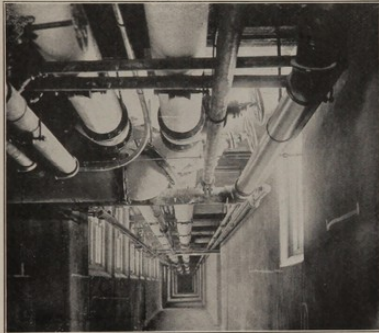
Fig. 14.—View in one of the cross tunnels.
