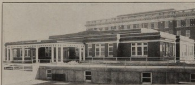
Fig. 17.—View of admitting department and out-door clinic.
