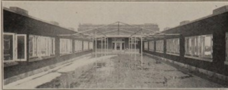
Fig. 13.—Roof garden on typical ward building (looking towards the head-house).
