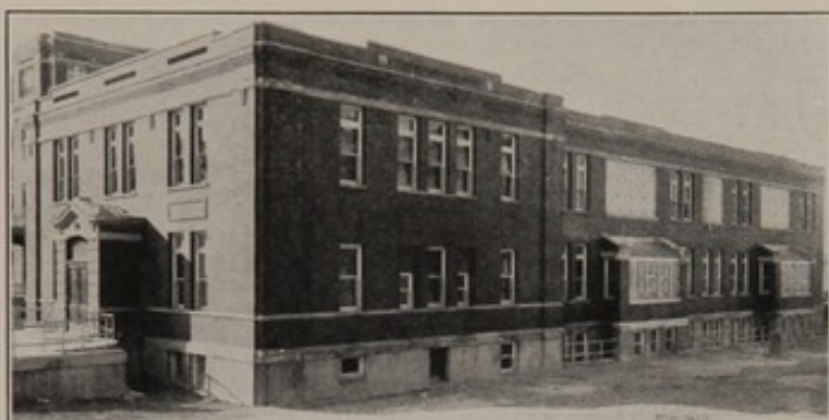
Fig. 16.—View of surgical pavilion.
