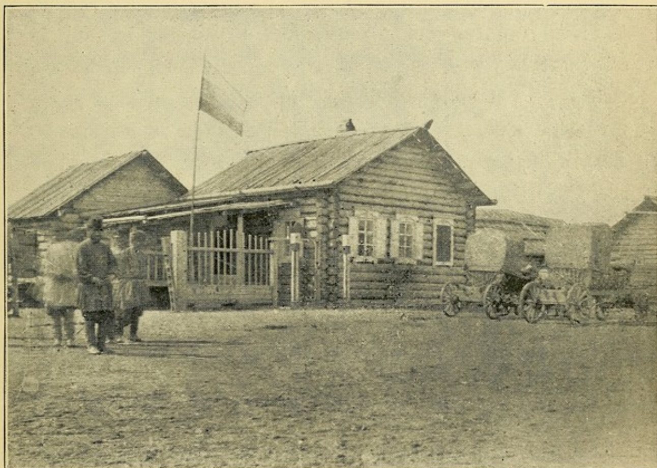
A POST-HOUSE STATION.
