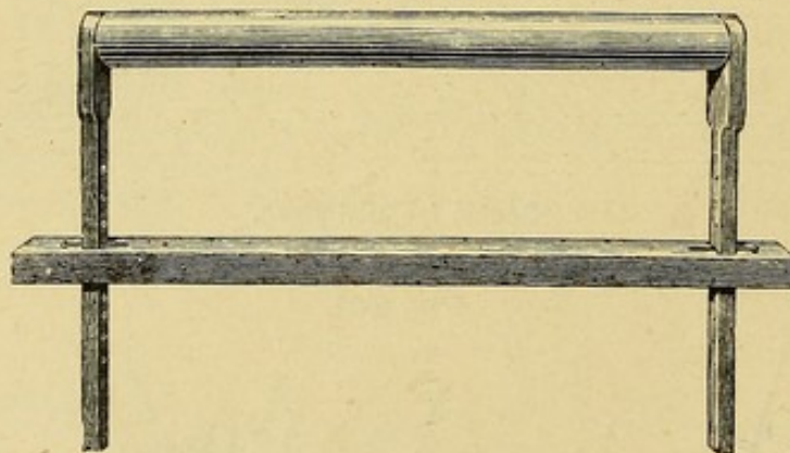
DOBSON'S wooden trestle for lifting the mattress.
