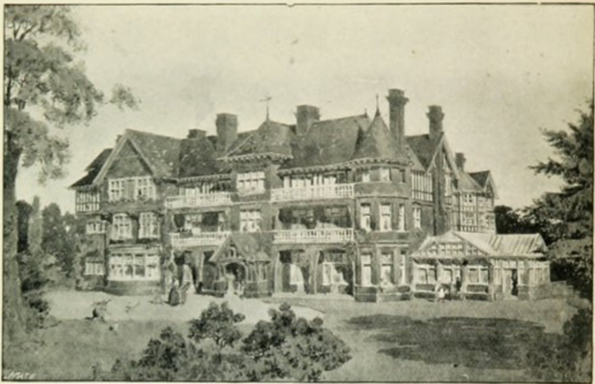
STOURFIELD PARK, BOURNEMOUTH ( front view ).
